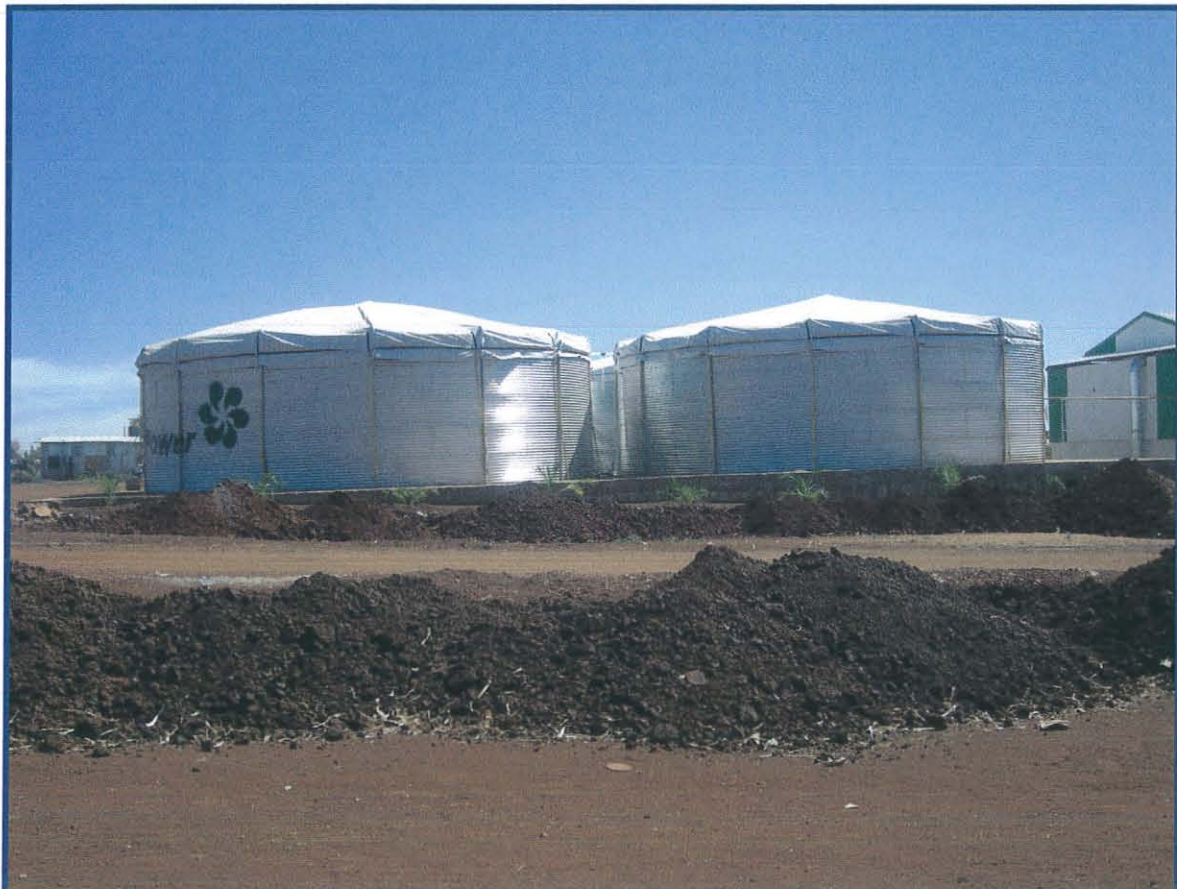
Picture 2: Oil Storage tank at the FloraEco Power's Factory in Fechatu
