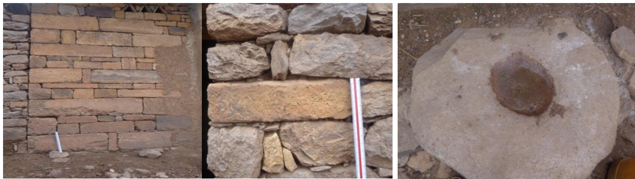
Fig.4.10: Comparison of architectural works (top left) dressed stones, (top middle) dressed stones bearing Sabeian inscription and (top right) circular slab with hole at the center all from Mai-Omo at the house of Merigeta Negash and (bottom left) dressed stones from Grat Be'al Gibri at Yeha.
