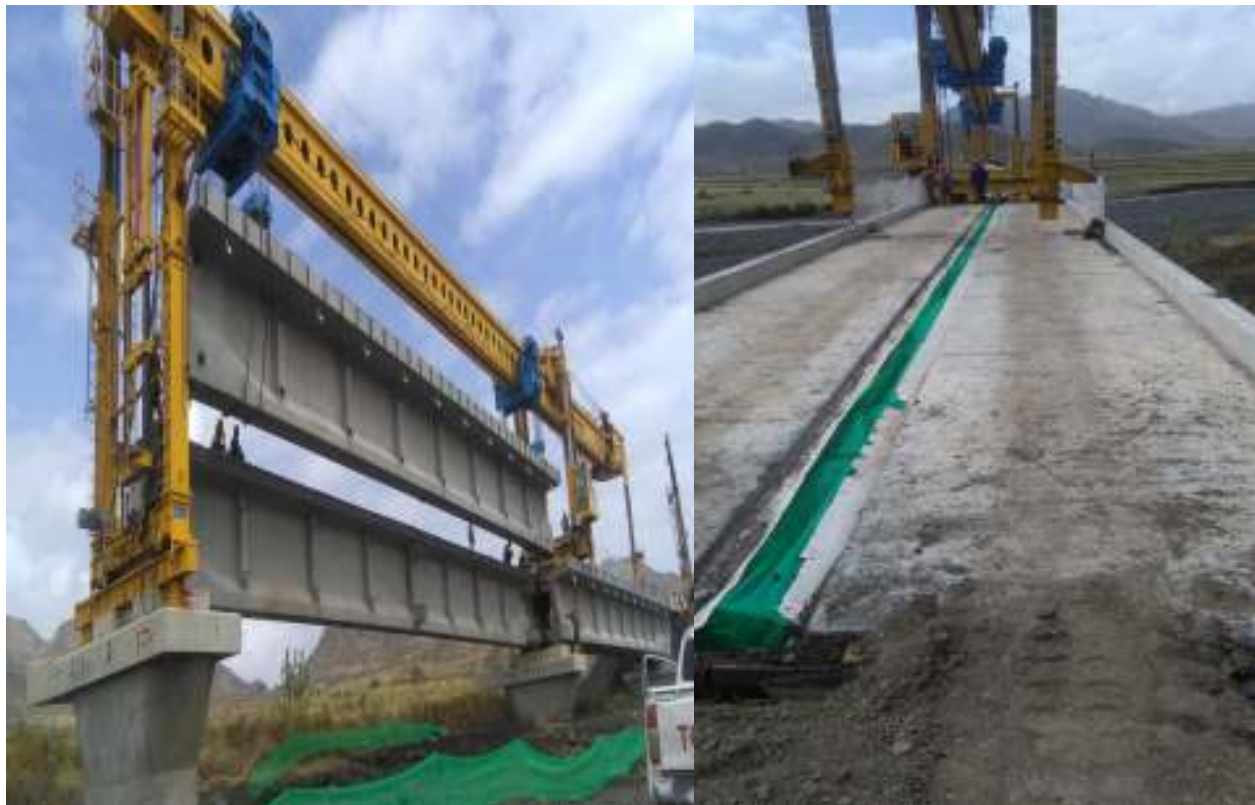
Figure 4-10: Erection of the bridge (On-site placement)
