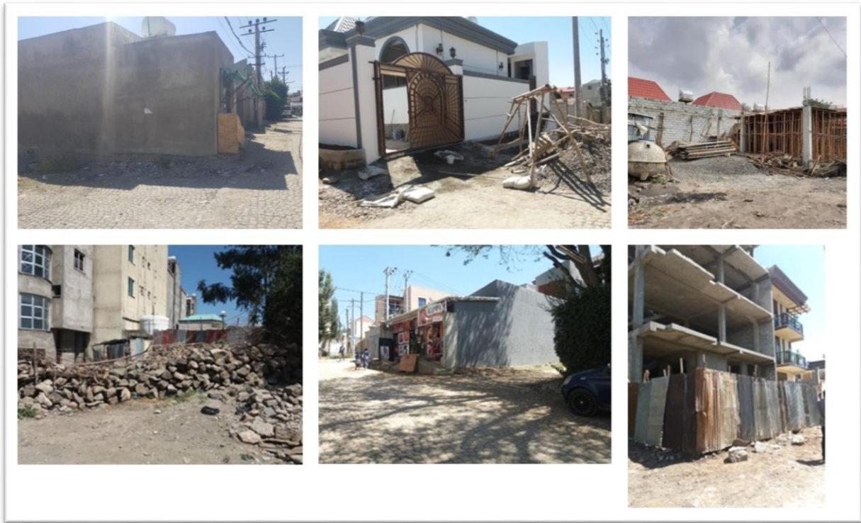
Figure 1: Green Area Violation in Woreda 12
