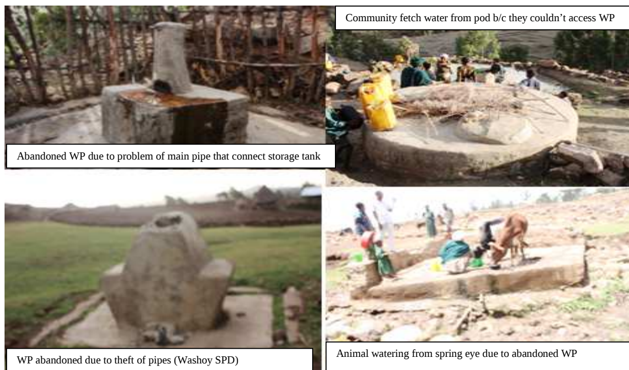
Figure 7: Abandoned spring developments
