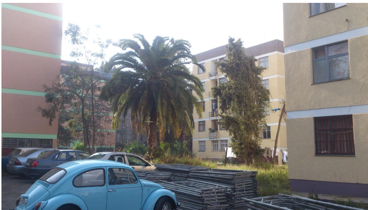
Fig. 5.10 external faced of the houses were repaired recently; see the scaffolding used for the maintenance work on the ground.
