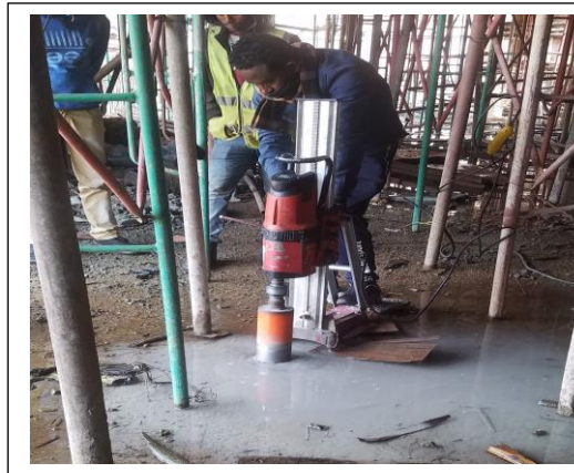
Figure 5.5. Core sampling (Pictured by researcher)
