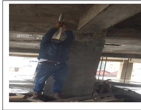
Rebound hammer reading from slab
