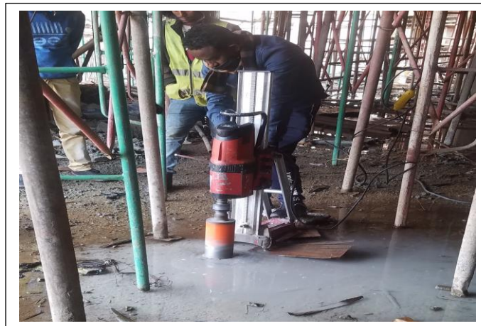
Concrete coring from floor slab
