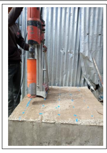
Casted slab and pad prepared for coring
