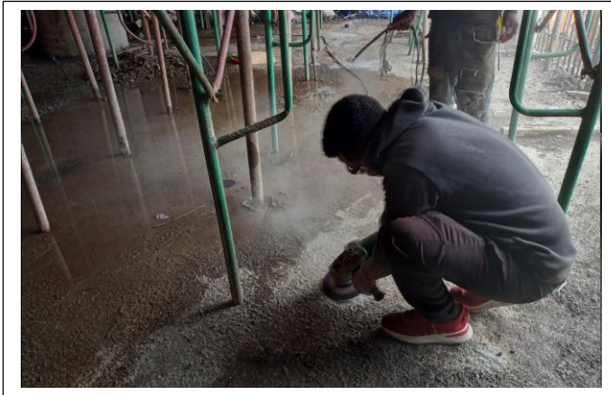
Slab surface polishing with grinder prepared for hammer
