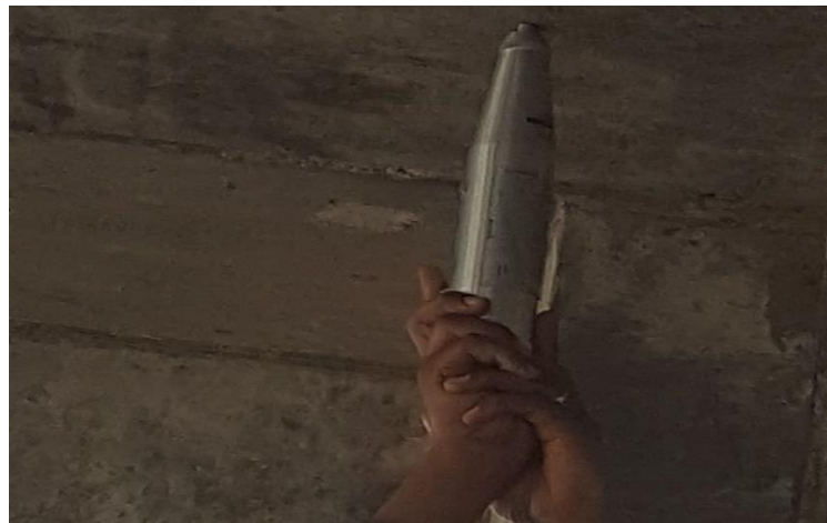
Figure 2.10. Schmidt Hammer test before the execution of the cores in an existing building.
