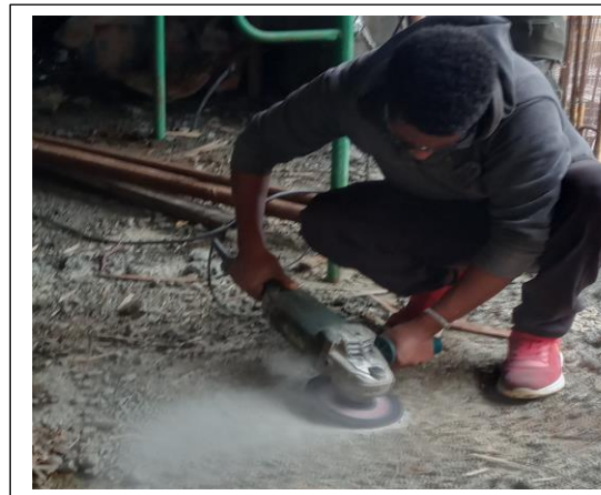
Figure 5.6. Surface preparation for hammer test on basement floor slab Fedengua site
