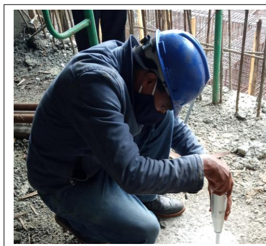
Figure 5.7. Conducting hammer test for basement floor slab Fedengua site
