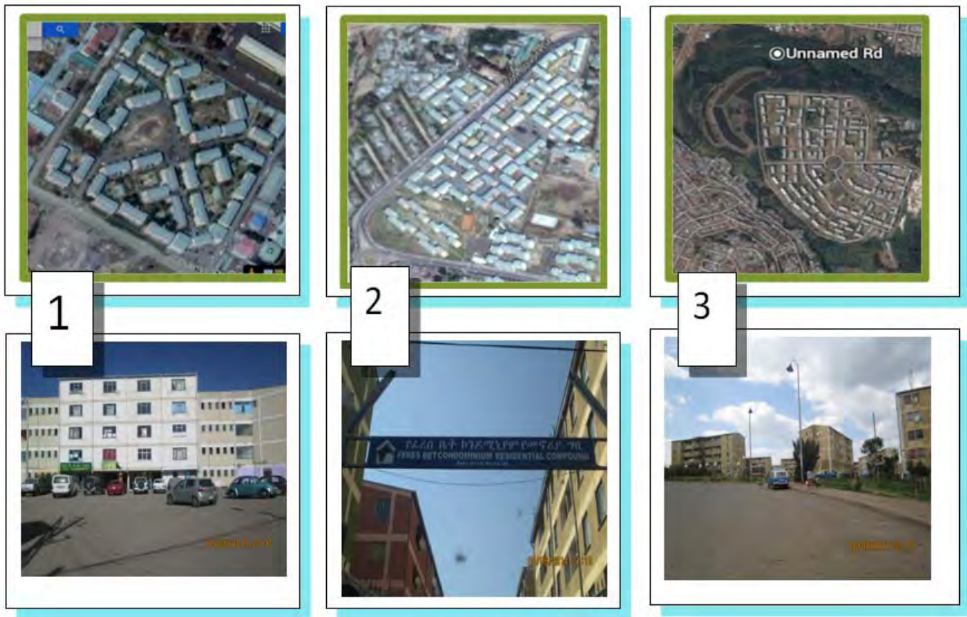
Figure 12: Three of the selected sites: the Bole Gerji, Feresbet, Mickey Leland respectively (Source: Google Maps [above]; pictures by author [beneath])
