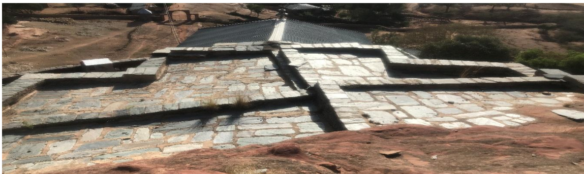
Figure 16: roof of the church.
