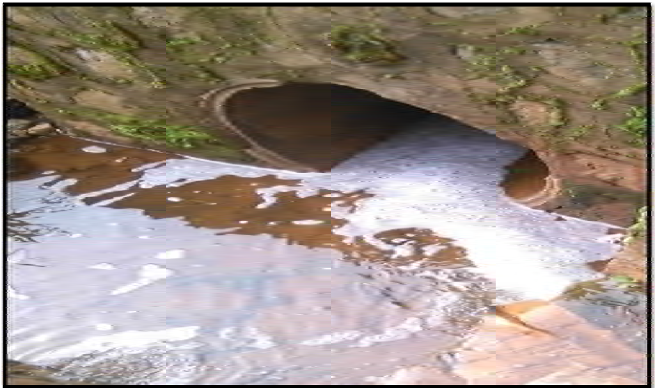
Figure 4.10: Drainage Structure (culvert) at Road Station 15+300
