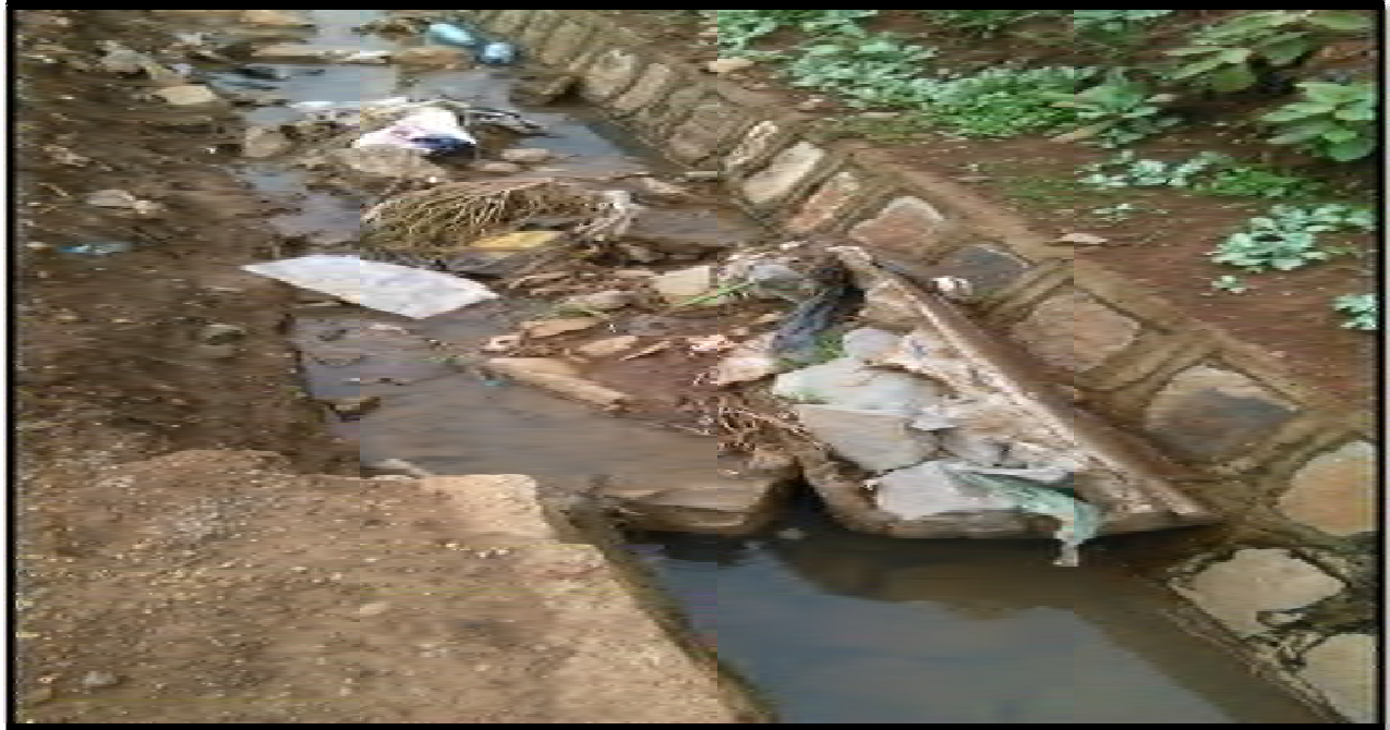
Figure 4.15: Road ditch at station 18+200
