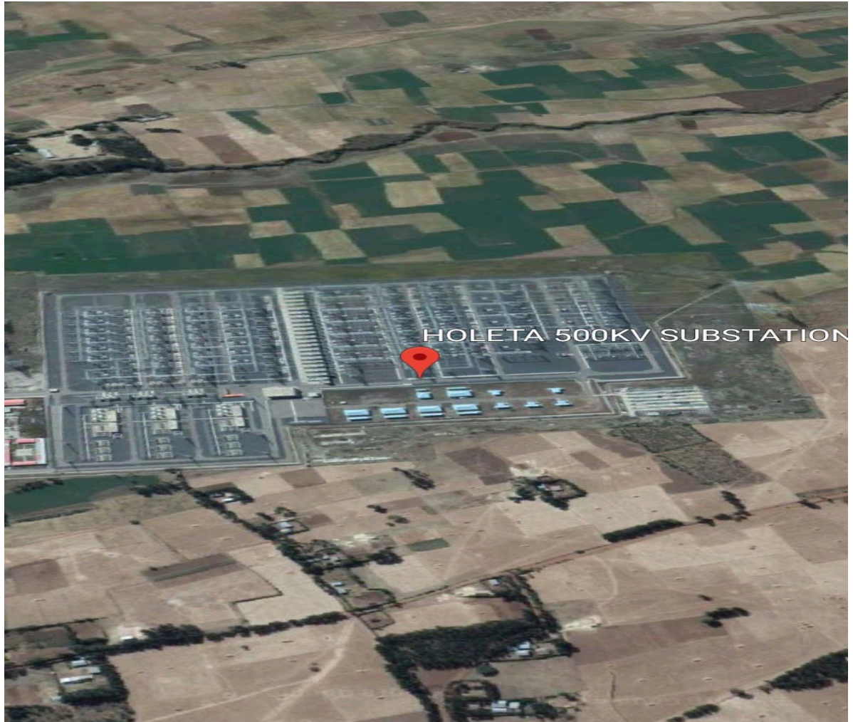
Figure 1.2: Google earth photo showing the substation switchyard and control room
