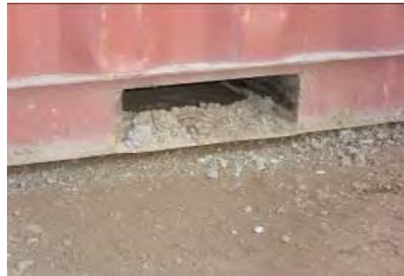
Figure 15: Mud in fork pocket [13]
