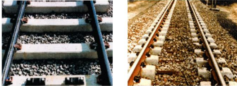
a) Mono block concrete sleeper b) Twin-block concrete sleeper
