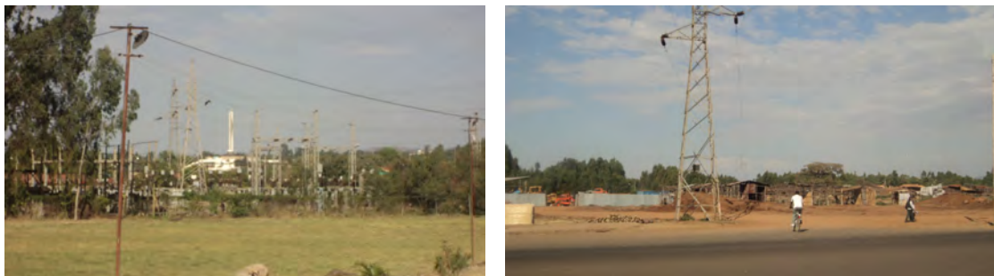
Source: Field survey (on December 2011), located inside Bahir Dar textile factory
