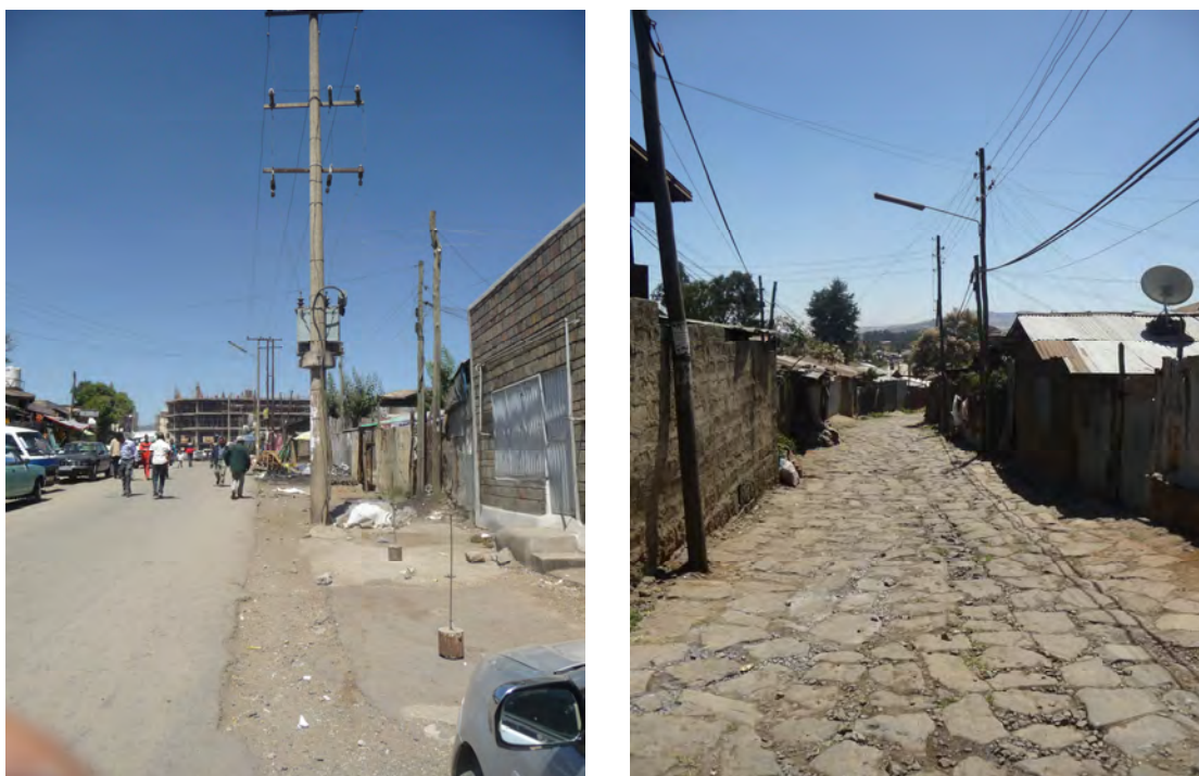
Figure 2.8: Shows the practice of an overhead electric system and poles installation in Addis Ababa City
