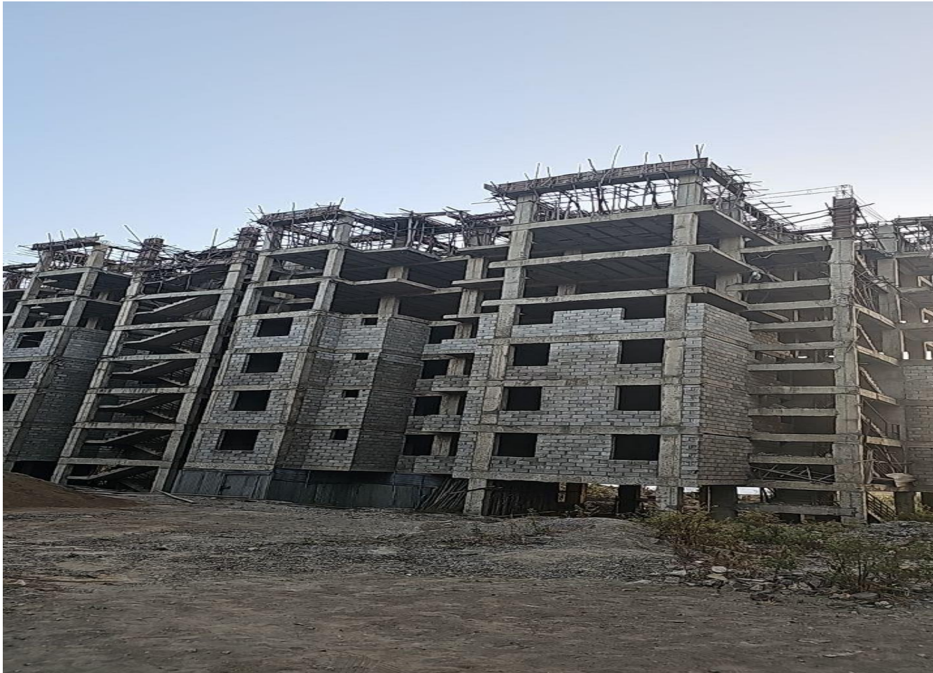
Figure 9 some of the blocks under construction in Furi Hana Site
