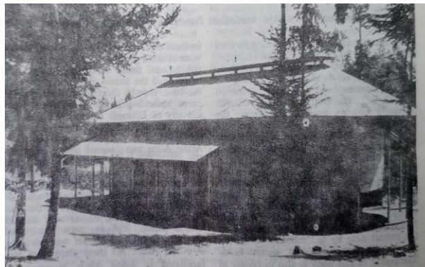
Figure 21 Old picture of the hall
