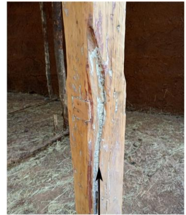
Consolidation using incompatible material
