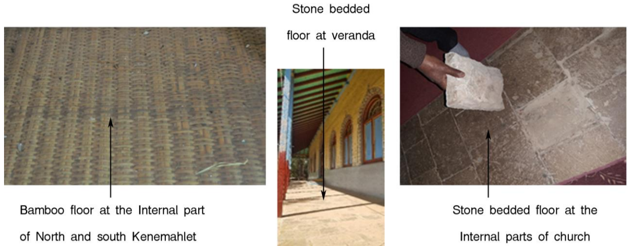
Figure 50 Condition of the church floor
