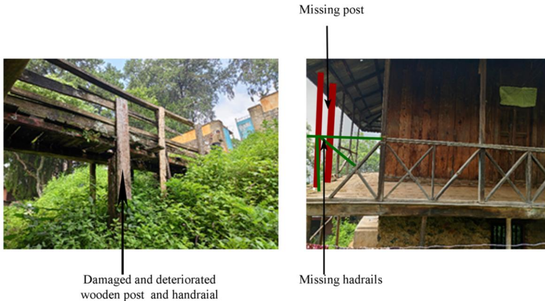
Figure 66 Condition of Nebirhood residence decorative details (handrail )
