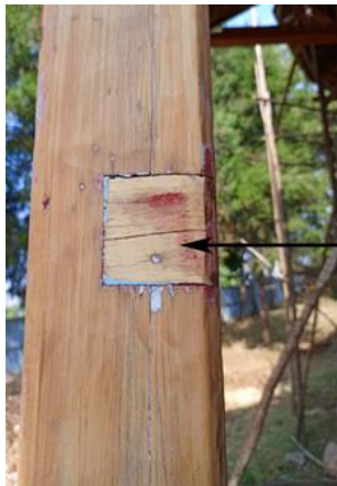
Figure 58 Pillars damaged by insects and termites
