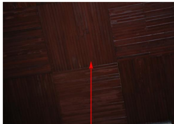
Wooden ceiling at the kedest of the church
