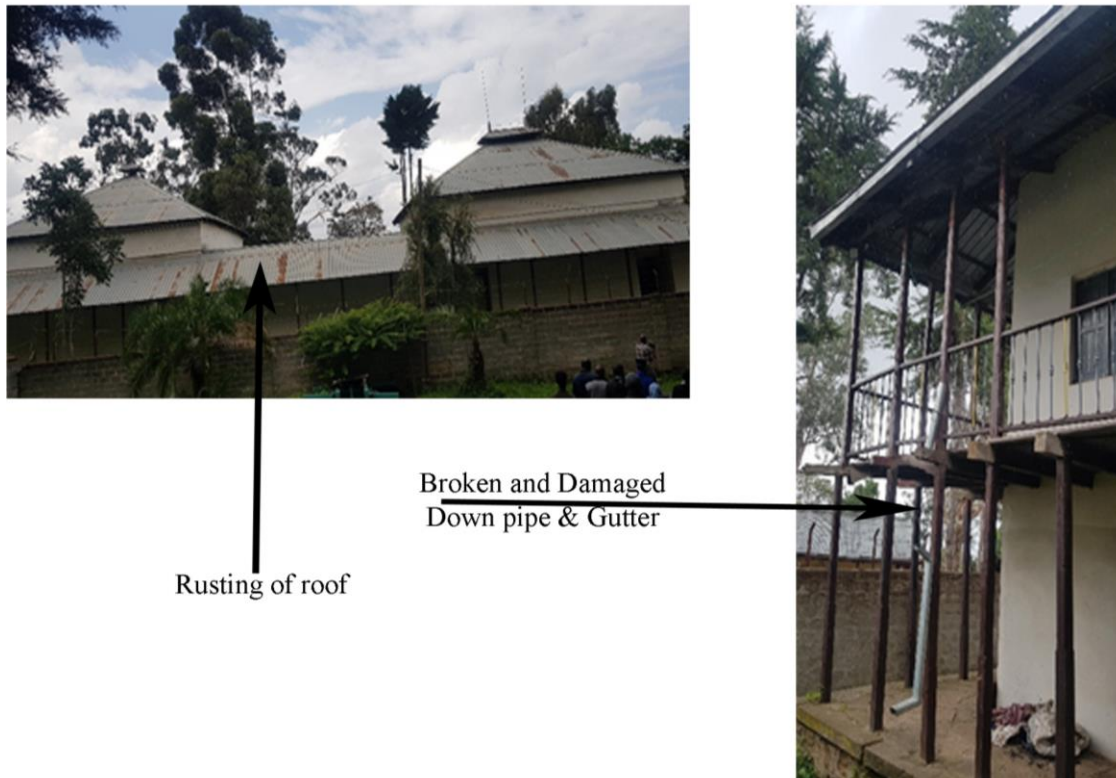
Figure 68 Current condition of roof
