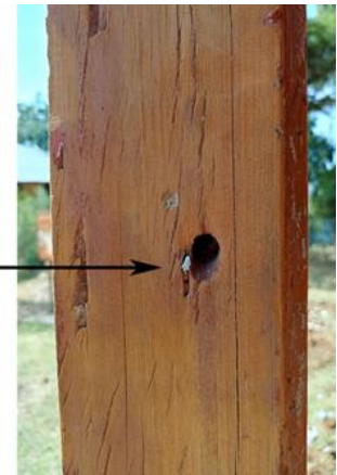
Consolidation using incompatible material
