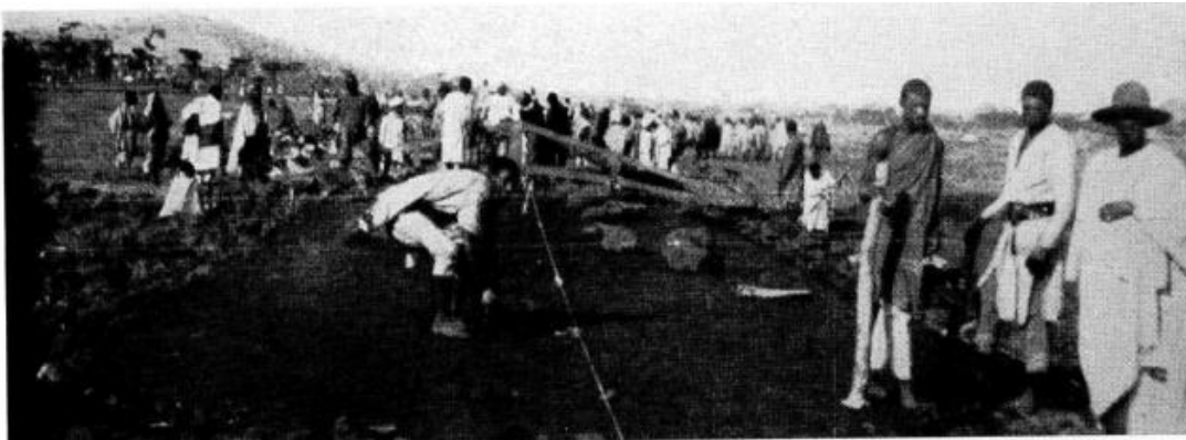
Figure 5 Road construction from Addis Ababa to Addis Alem
