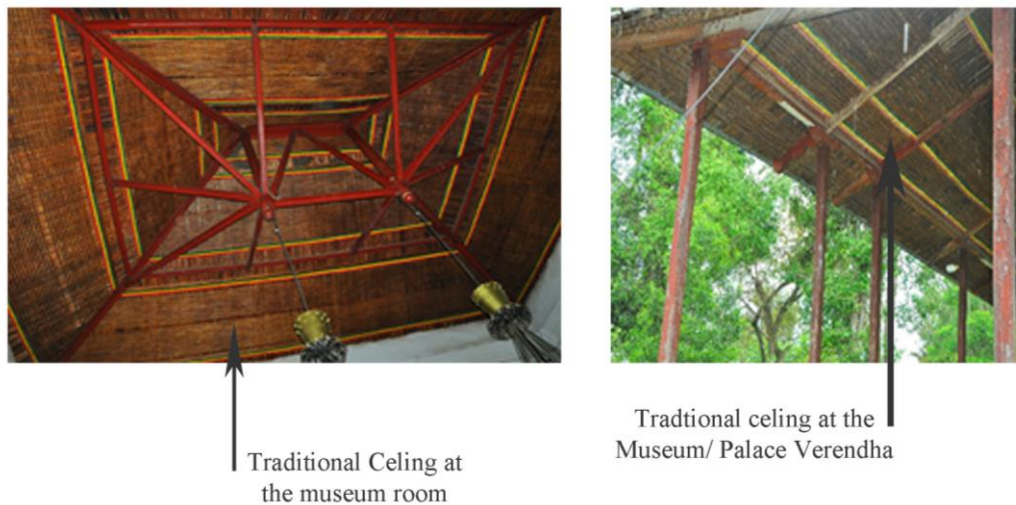
Figure 70 Ceiling current condition of palace ceiling
