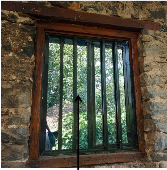
Wood window change into glass and steel
