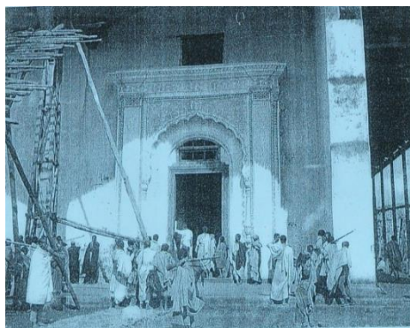
Figure 2 During the construction of the church in 1900
