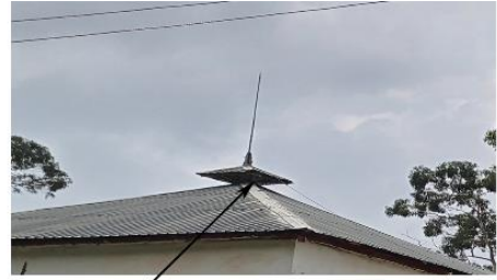
Finials at the roof top parts
