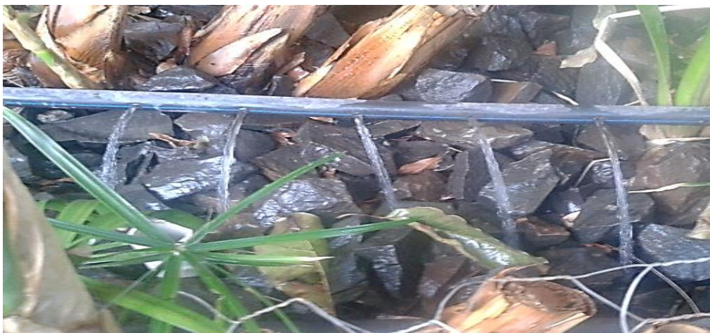
Figure 8. Influent distribution of the Pilot VSSFCW
