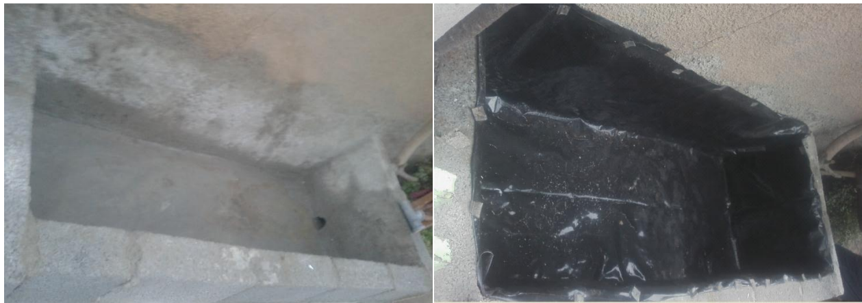
Figure 3. Plastered and impermeable plastic cover of pilot plant
