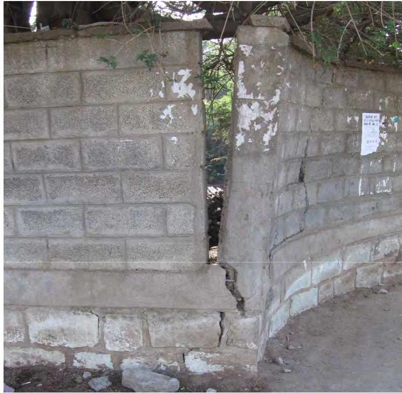
Figure 2.3.2 Failure of fence [2]
