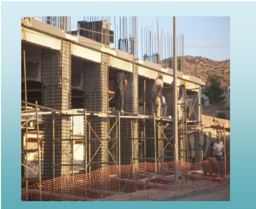
Figure 14: Concrete Jacketing in practice
