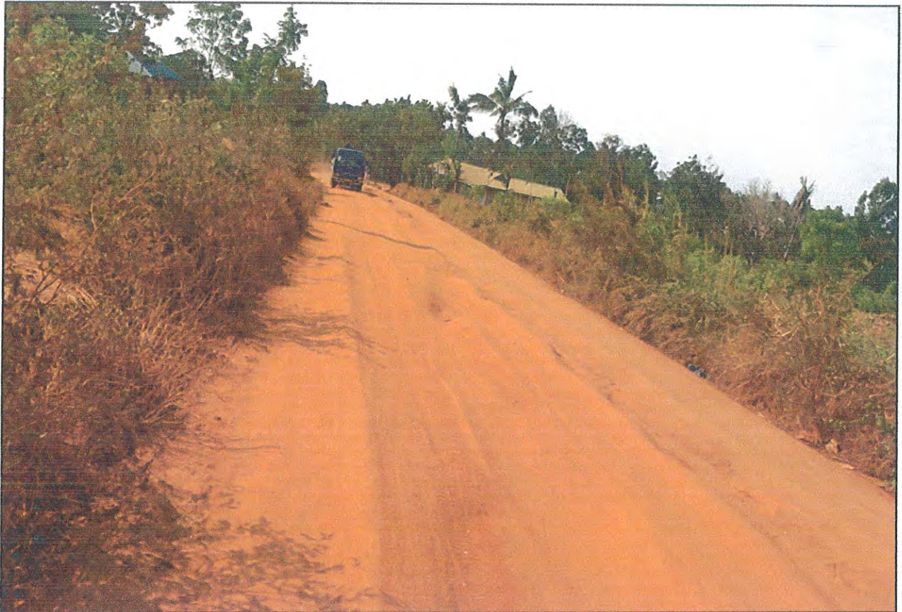
Figure 6.2 Earth road connecting Msumi sub-ward to the trunk road (Morogoro road)
