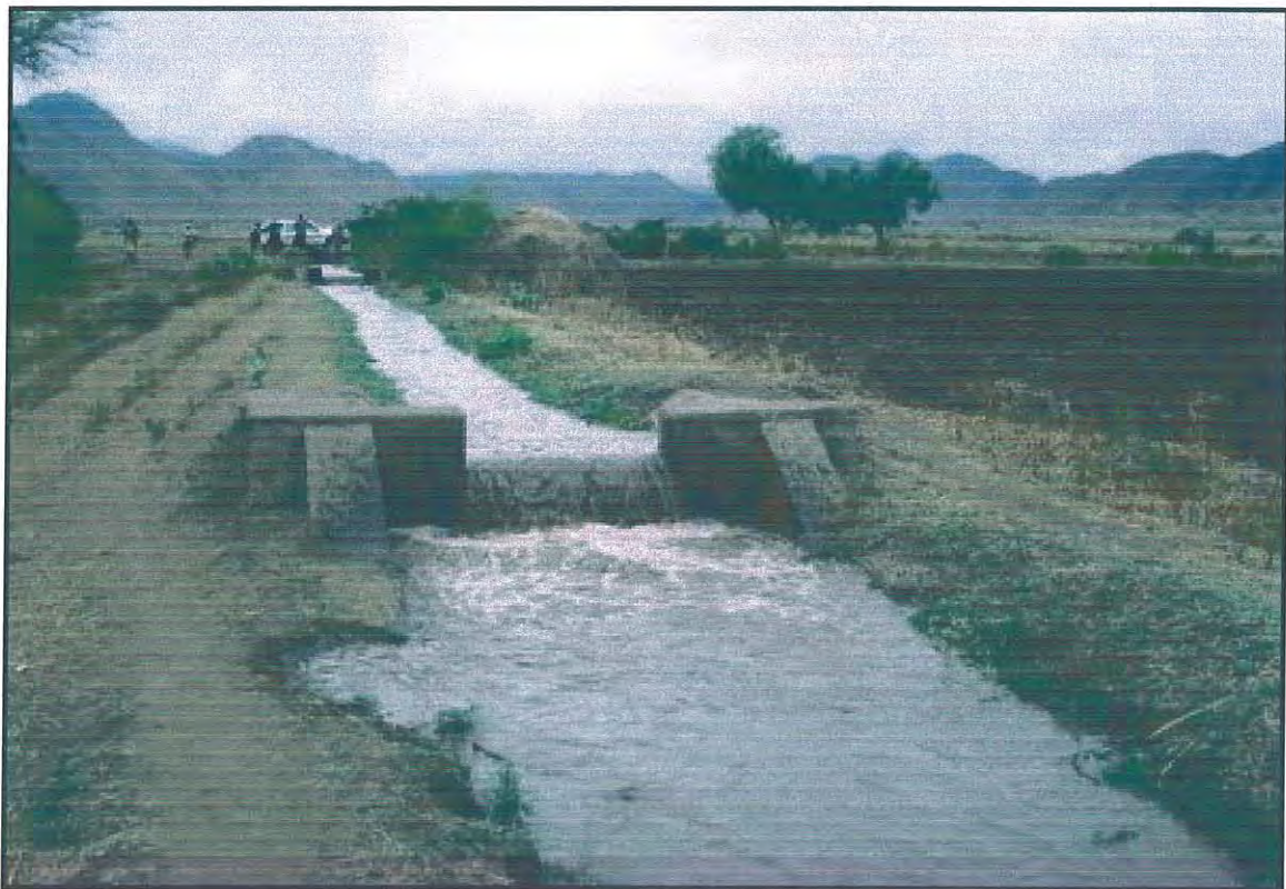
Figure 6 Alawuha irrigation primary canal
