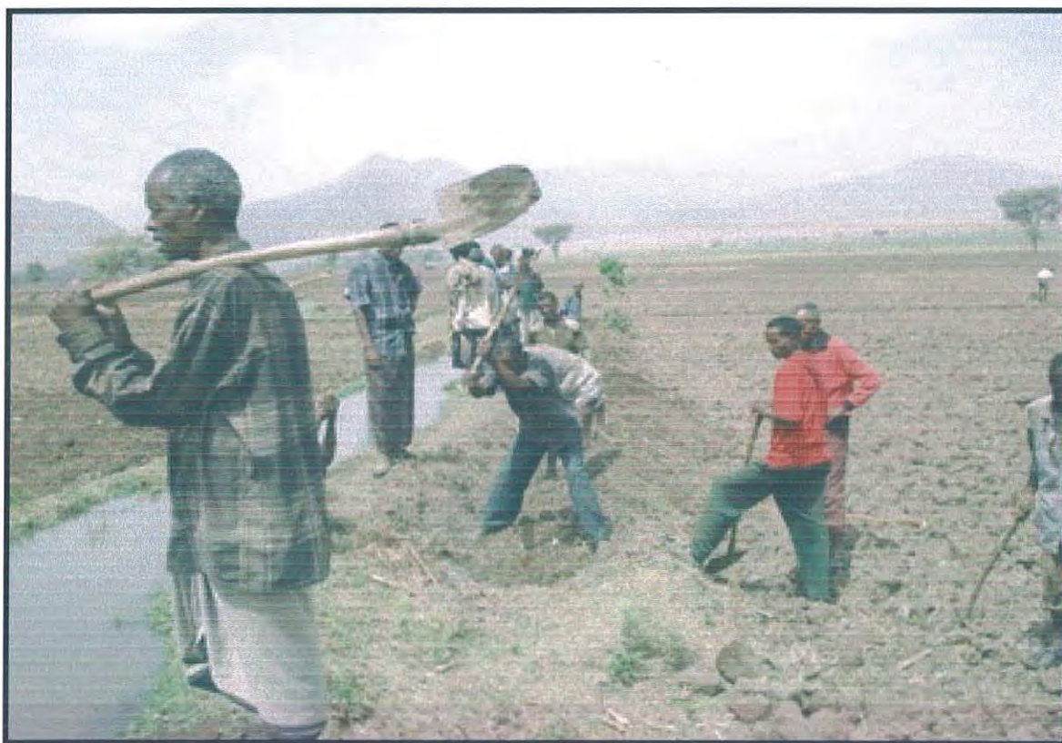
Figure 5 Community maintenance work at irrigation canal
