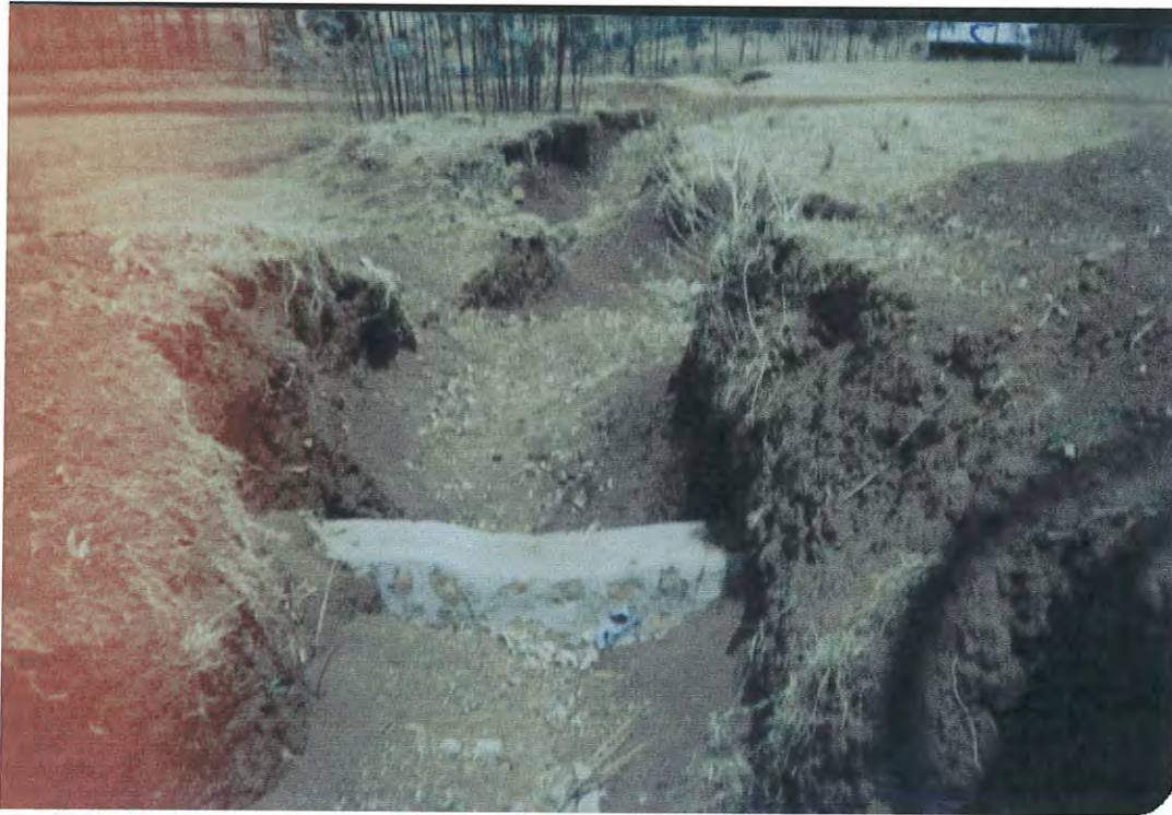
(Photo 7.1a): A modern check dam in Mellit village (Photo: By the researcher)
