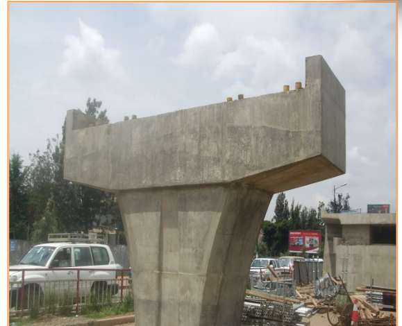
Fig. 2.4: Tapered column used in Addis Ababa railway systems
