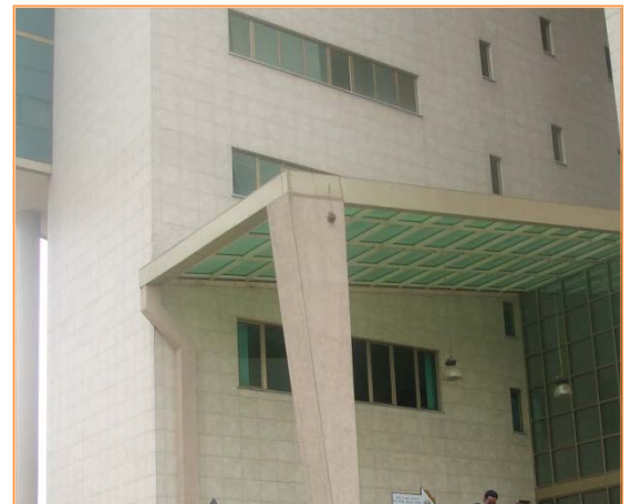
Fig. 2.5: Tapered column used in head office of Awash international bank, Addis Ababa
