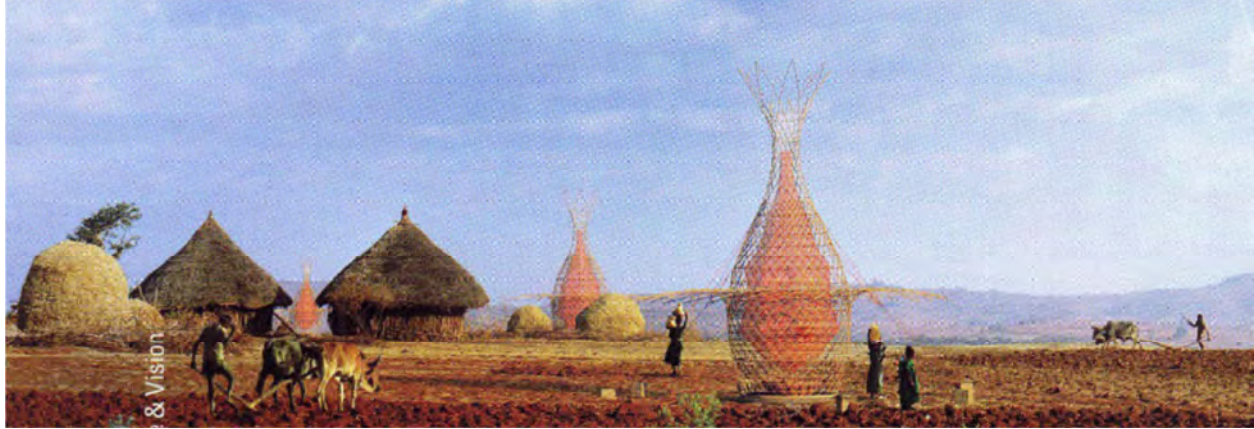
Figure 3-3 Warka water project: water collecting modules
