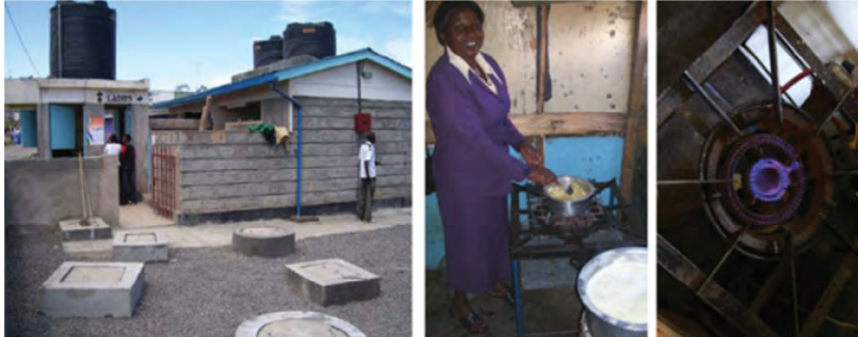
Figure 3-4 Lavatory and Wastewater Treatment Plant with Installed Biogas Generation Facility
