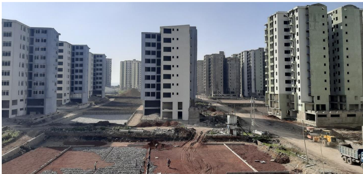
Figure 4.6. Partial External view of Bole Beshale project site buildings
