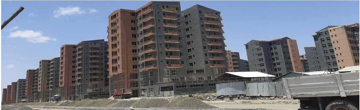
Figure 4.4. Currnt external view of Bole Ayat-1 project site
