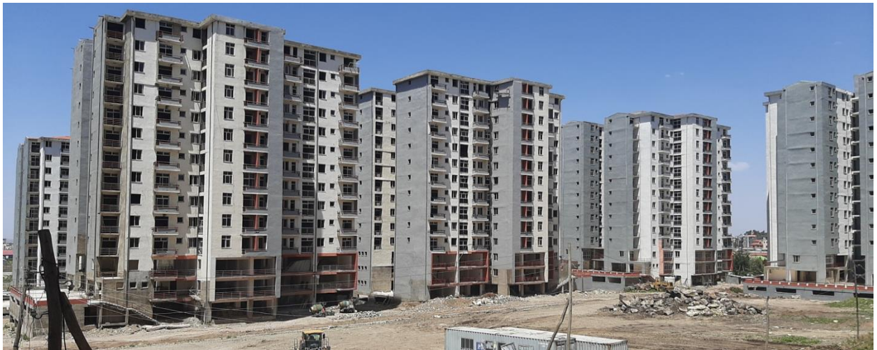
Figure 4.5. External view of 2B+G +13 typology Meri site buildings
