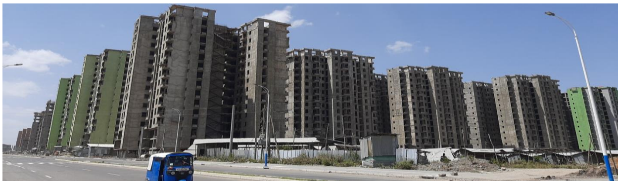
Figure 4.10. Partial External view of Bole Ayat-2 project site-2
