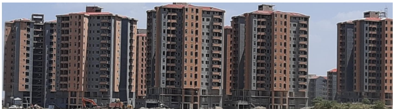
Figure 4.13. Partial External view of Bole Ayat-2 project site-4
