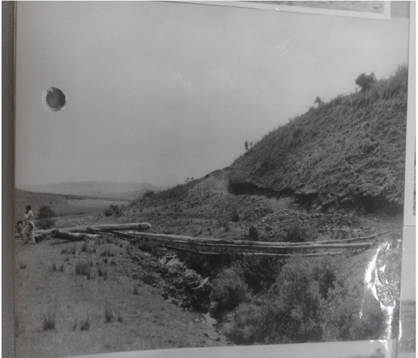
Figure 4: 2 Traditional Bridge in the Study Area (1962)
