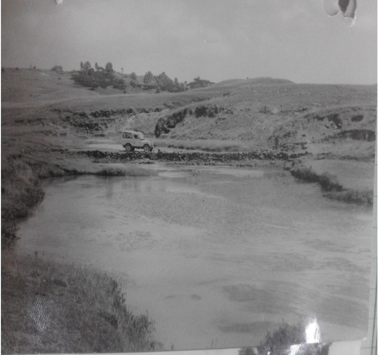
Sanford's Report on the improvement of transportation in the wäräda , in the early 1960s
