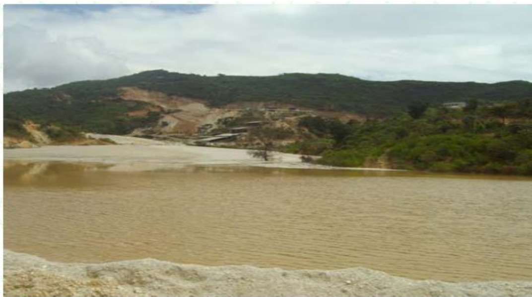
Figure 3.1.5-2: tailing dam of tantalum ore washing site.
