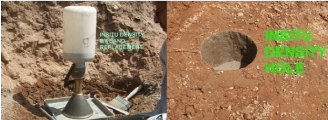
Figure 4.1.3 In situ density test of concrete pre-cast for conditioning (treatment).
