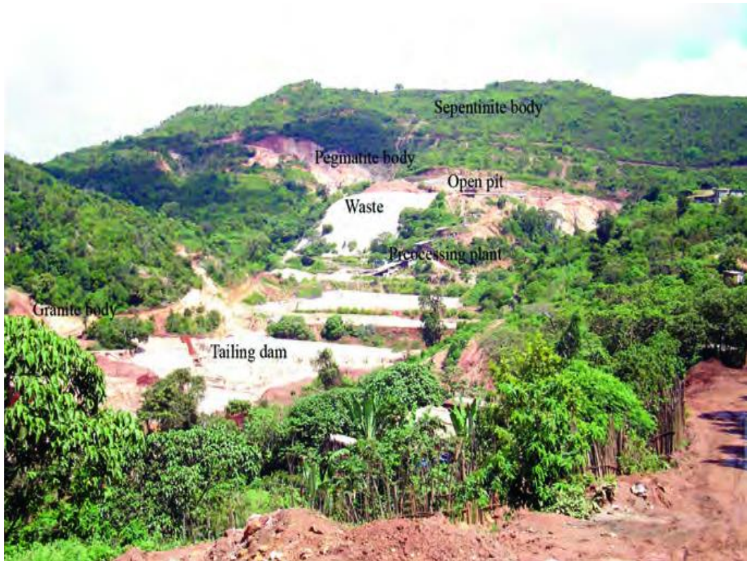
Figure 1.1-1: Topography of Kenticha tantalum open pit mining site (MME, 2010)
