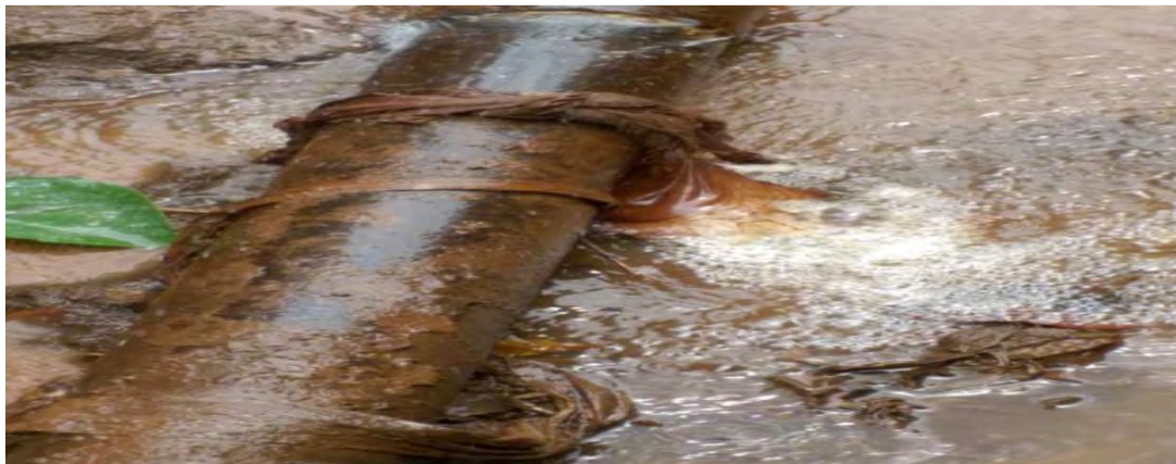
Photo from Water line and sewerage system in Dila Twon July 2016
