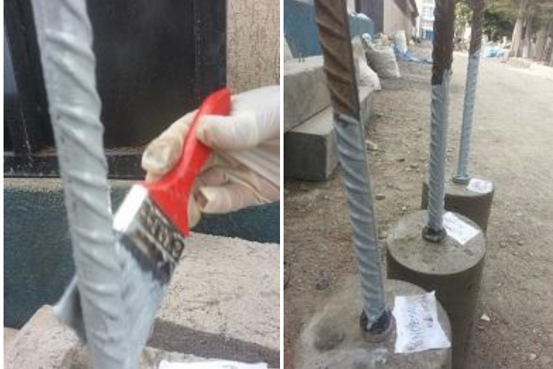
Fig. 3.10 Application of Anti-corrosion paint
