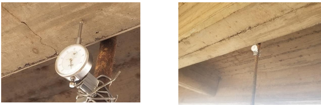
Figure 3.12: Deflection measuring gauge, installed at the mid of the first span of Koka river bridge
