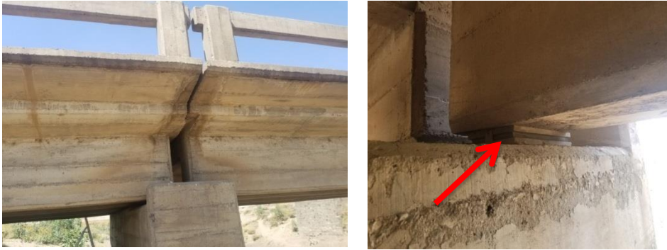
Figure 3. 2: Bridge support, Elastomeric bearing
