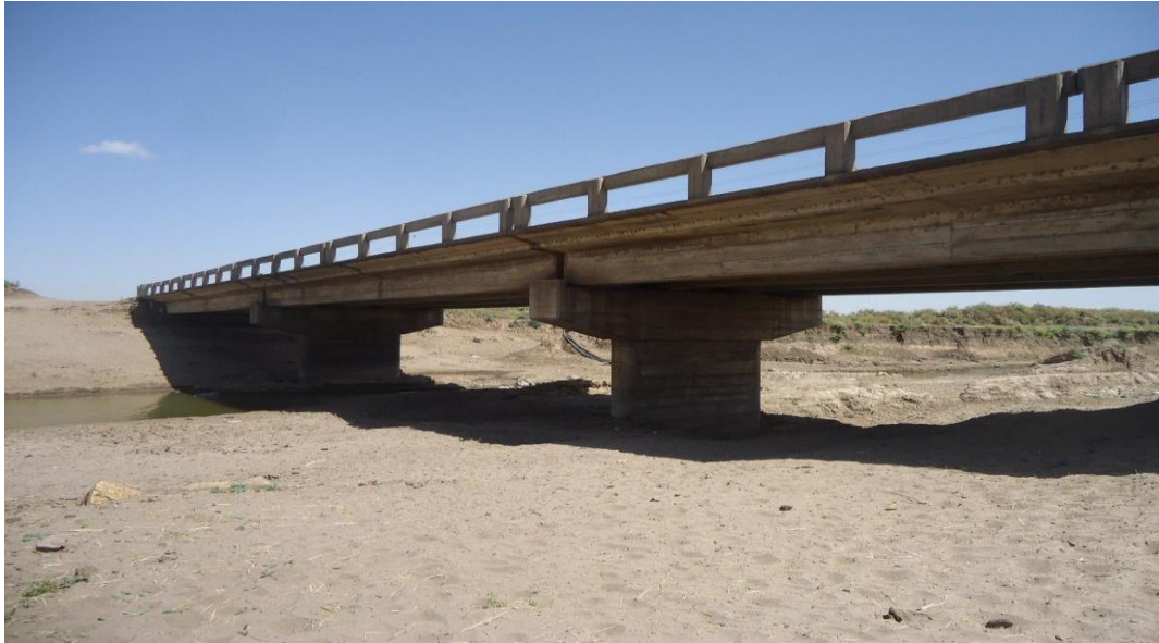
Figure 3. 1: Koka river bridge
