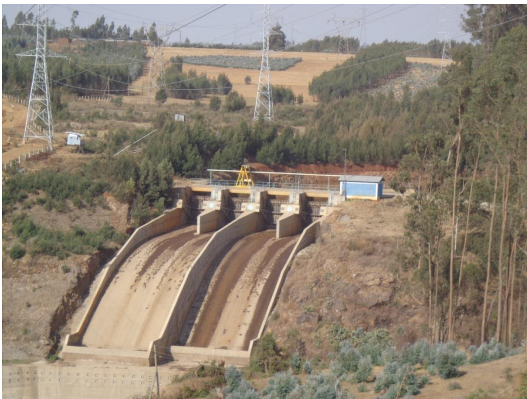
Plate 2.1 Gefersa dam - one of the main dams that supply drinking water to Addis Ababa
