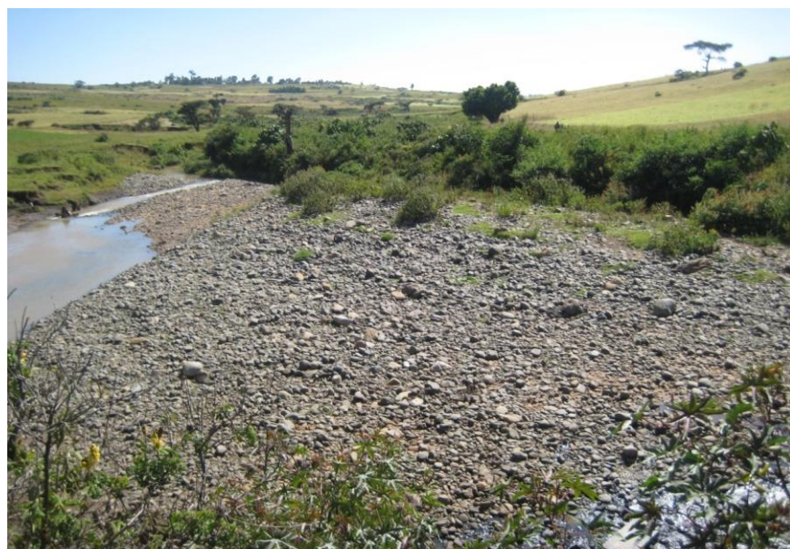
Plate 5.5 Area 1 - Proposed Shell and Filter material at the downstream of the Berga River
