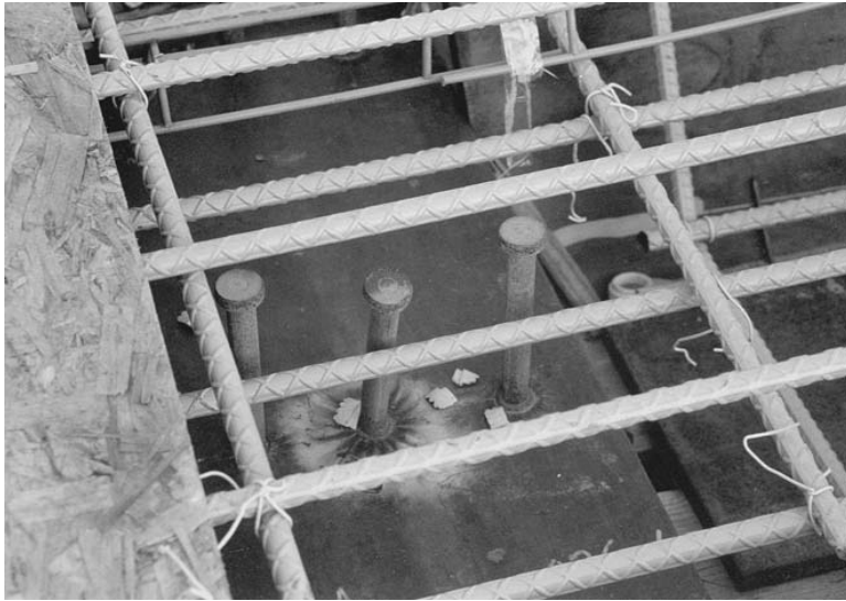
Figure 2.13: A shear stud installed at the top flange of a plate girder.
