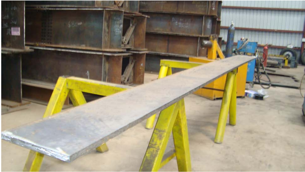
Plate 3.2: Metal sheet ready to manufacture I profile plate girder for steel bridge.
