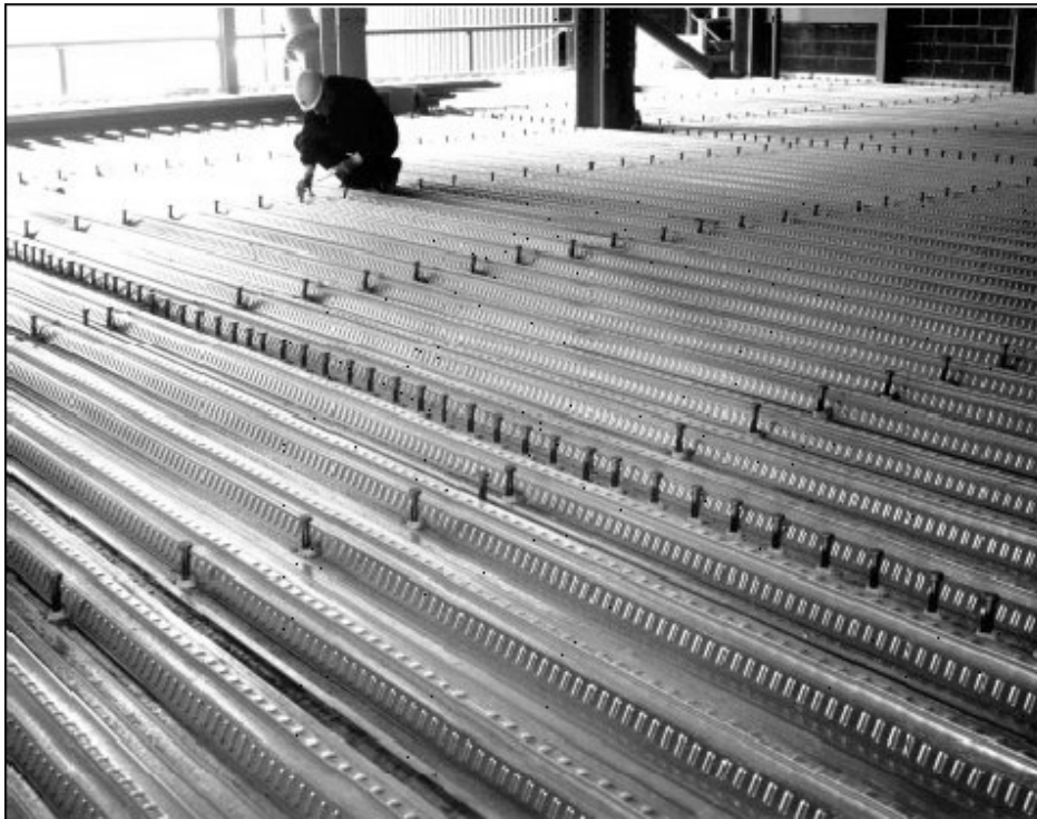
Figure 2.1: Use of metal decking
