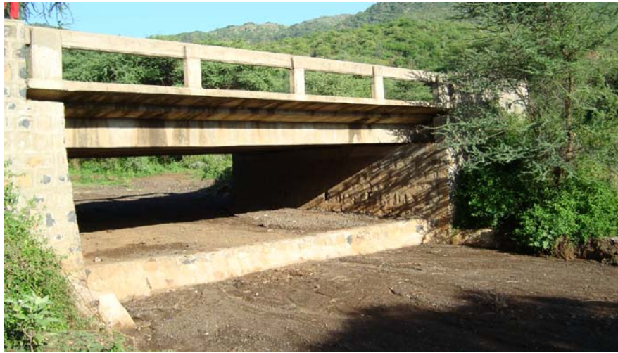
Plate 3.5: Reinforced concrete deck girder bridge
