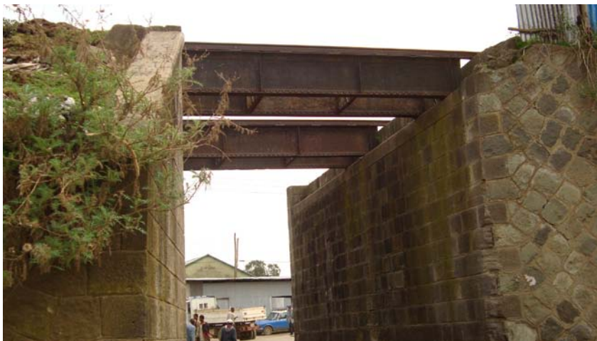
Plate 3.7: Steel bridge in railway for train passage
