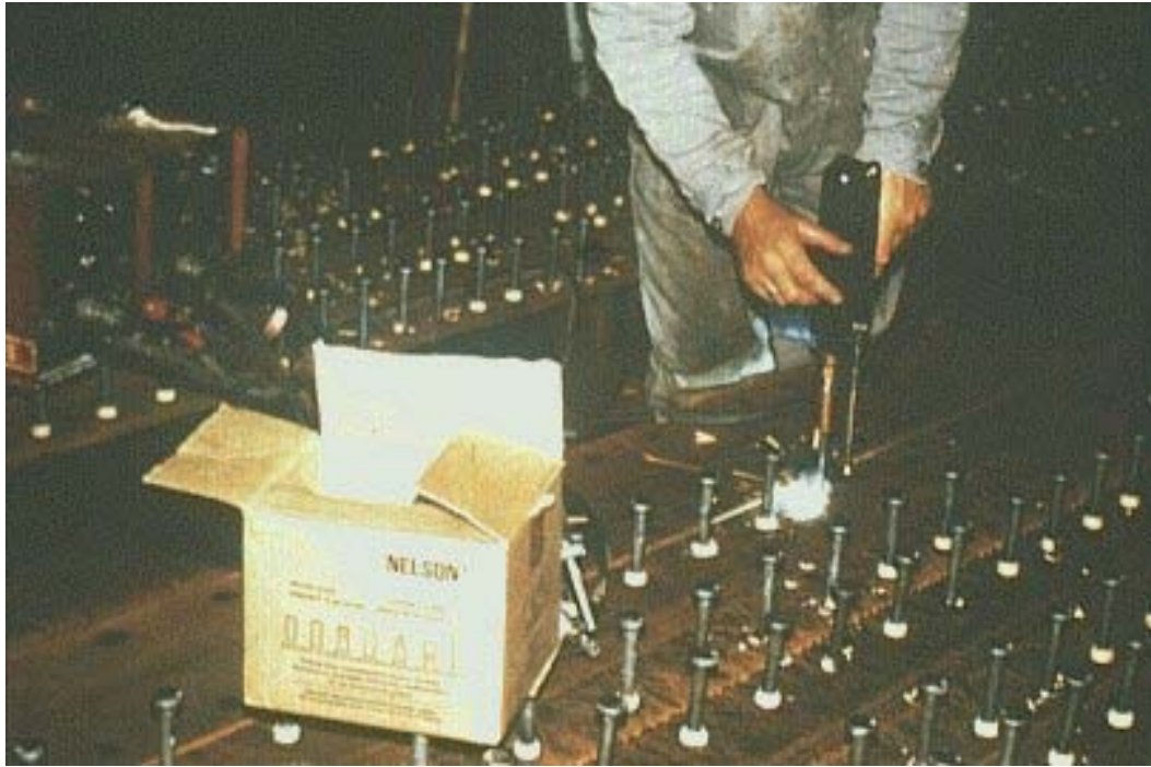
Figure 2.14: Shear studs being welded on steel beam flange
