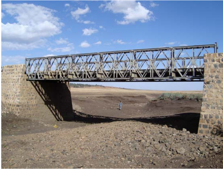
Plate 3.6: Bailey bridge being used as temporary passage (detour)
