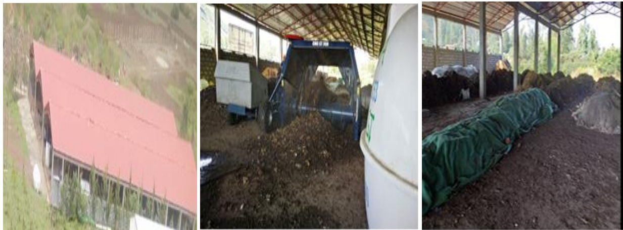
Figure 5. Current compost plant of Bishoftu city
