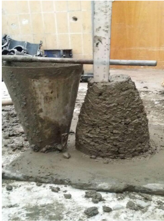
Figure 4-2: Slump test for fresh concrete
