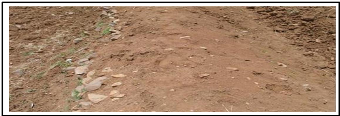
Figure 4.3. Stone faced soil bund structure of the study area
