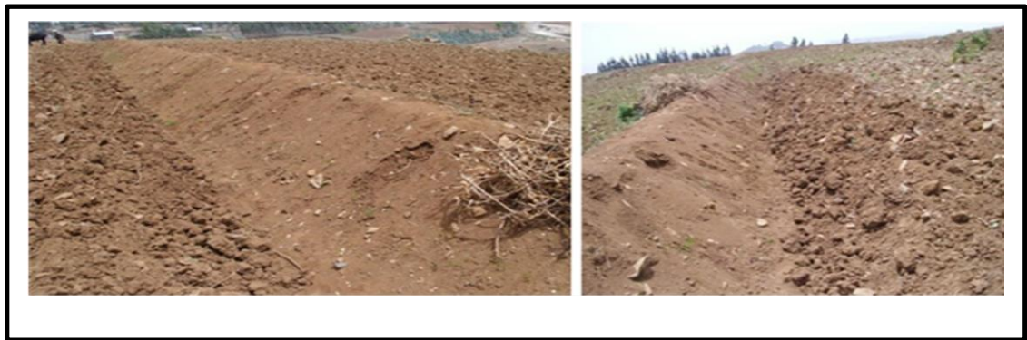
Figure 4.6 soil bund of the study area
