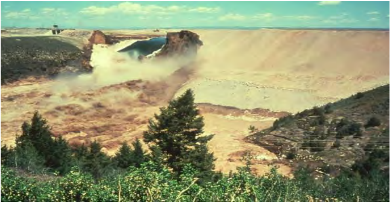
Figure 2.2: Teton Dam failure, Rexburg, ID, June 1976
