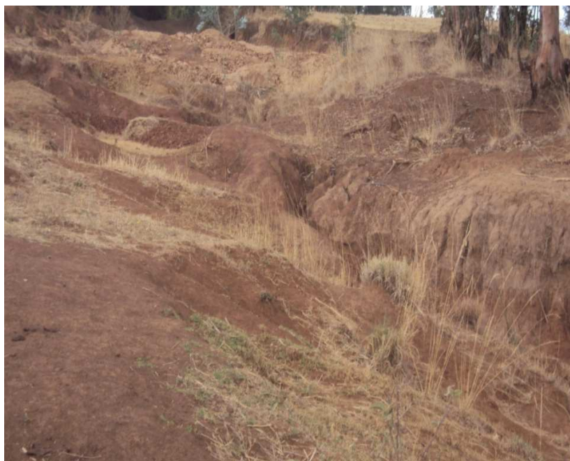
Figure 4.7: Gully formation in Hayise kebele ( photo by the researcher; February, 2015 )
