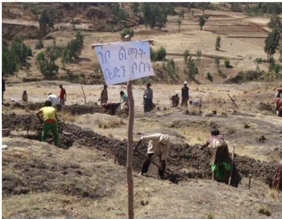
Figure 4. 6: Gully rehabilitation by structural methods in Belessa kebele (Photo by the researcher, February, 2015).
