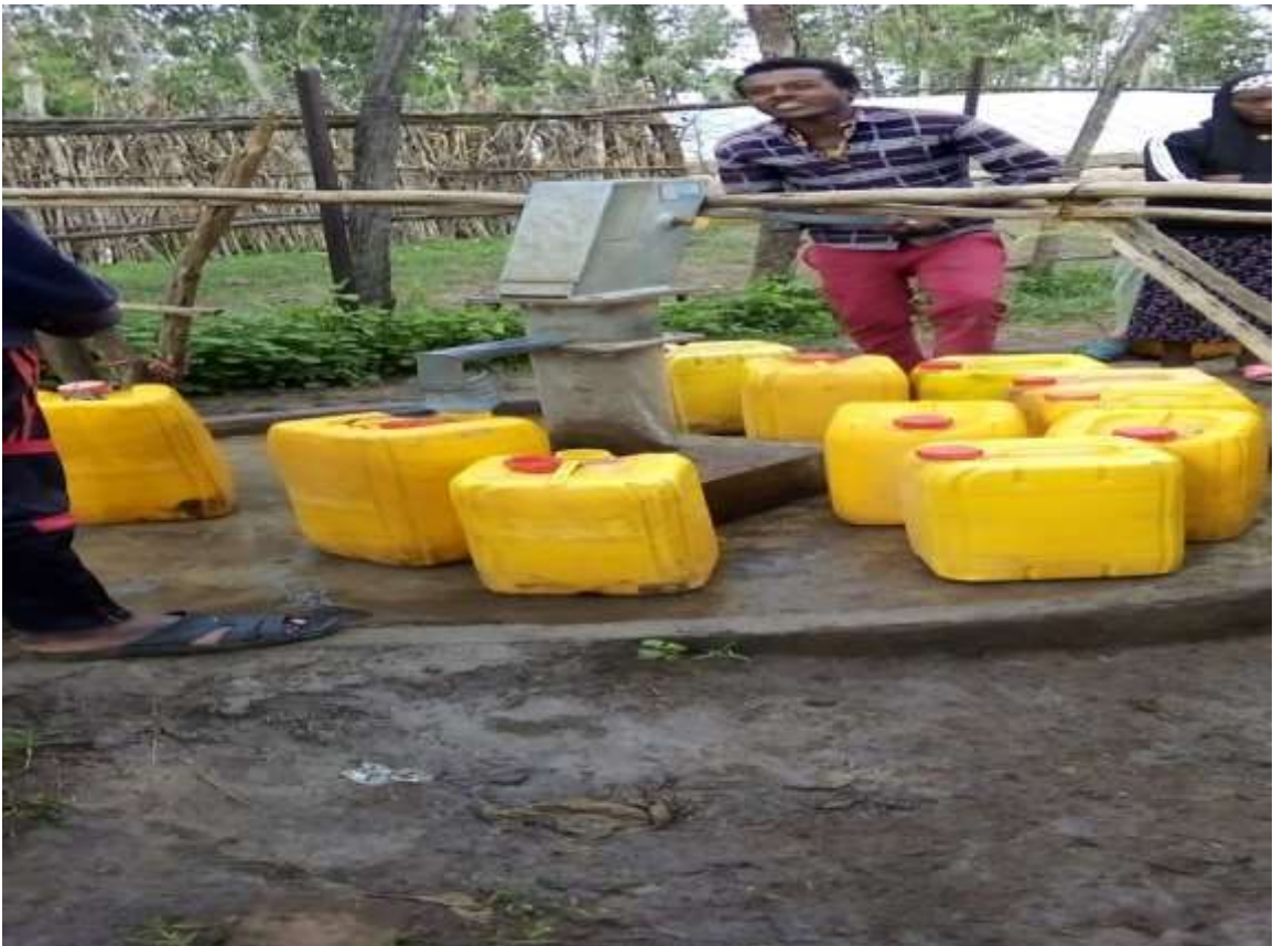
Figure 6: The presence of fence as protection system of Water scheme
