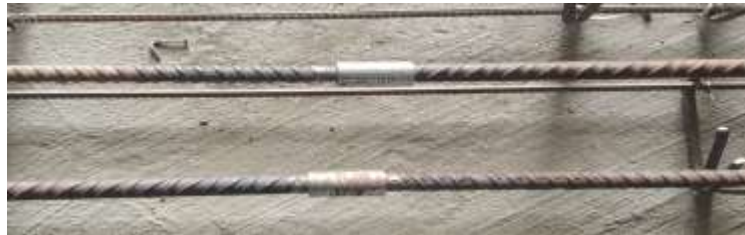
Figure 3-4: Photography of Coupler Connected Reinforcement Specimen
