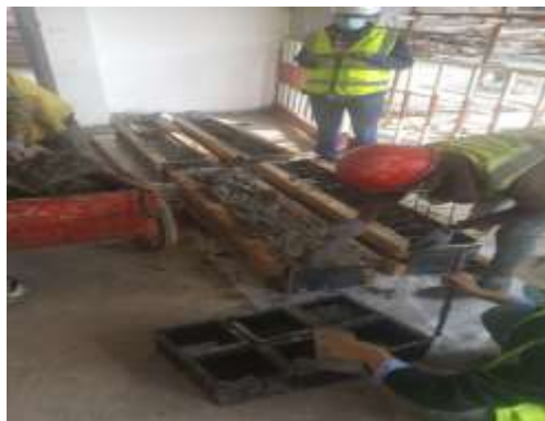
(a) Fresh Concrete Pouring
