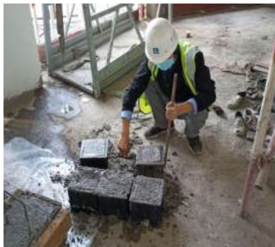
Figure 1D: Cube Strength Test Sampling
