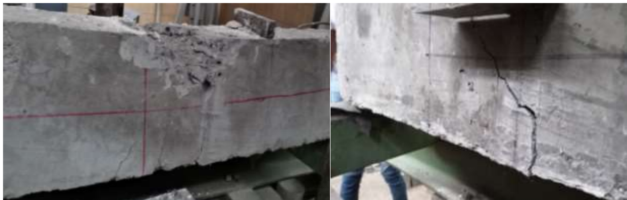
1. Cracking Behavior of B1
