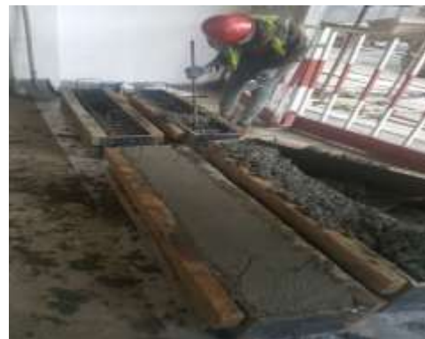
(b) Compacting in the Mold
