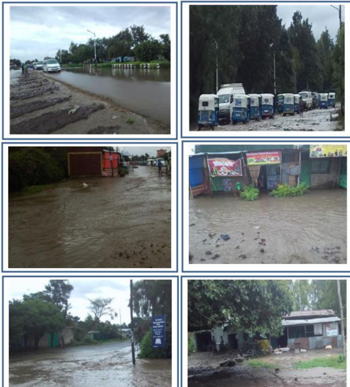
Figure 2. Overflow of drains nearby Ethio-Japan Textile Factory (8:30 AM, July 15/2020)
