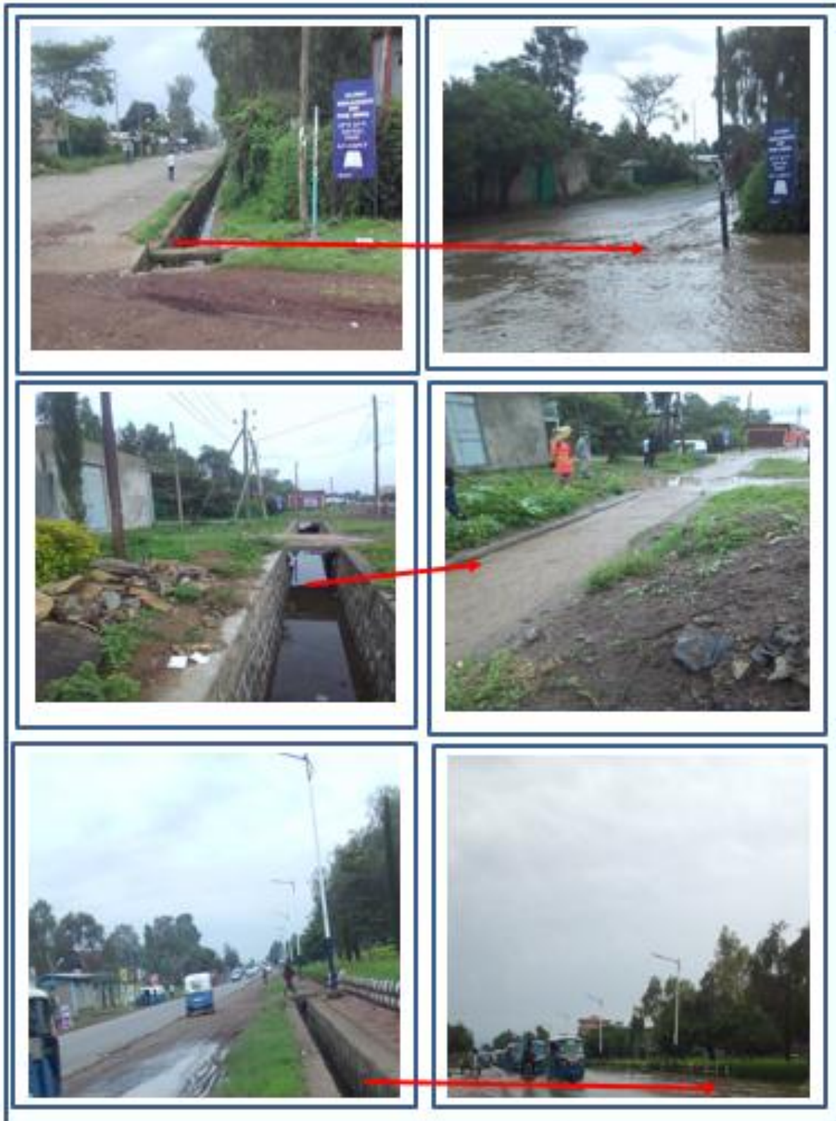
Figure 40. Pictures of drains before & at the moment of flooding.
