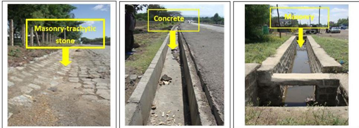
Figure 13. Some pictures of drainage infrastructures of the town
