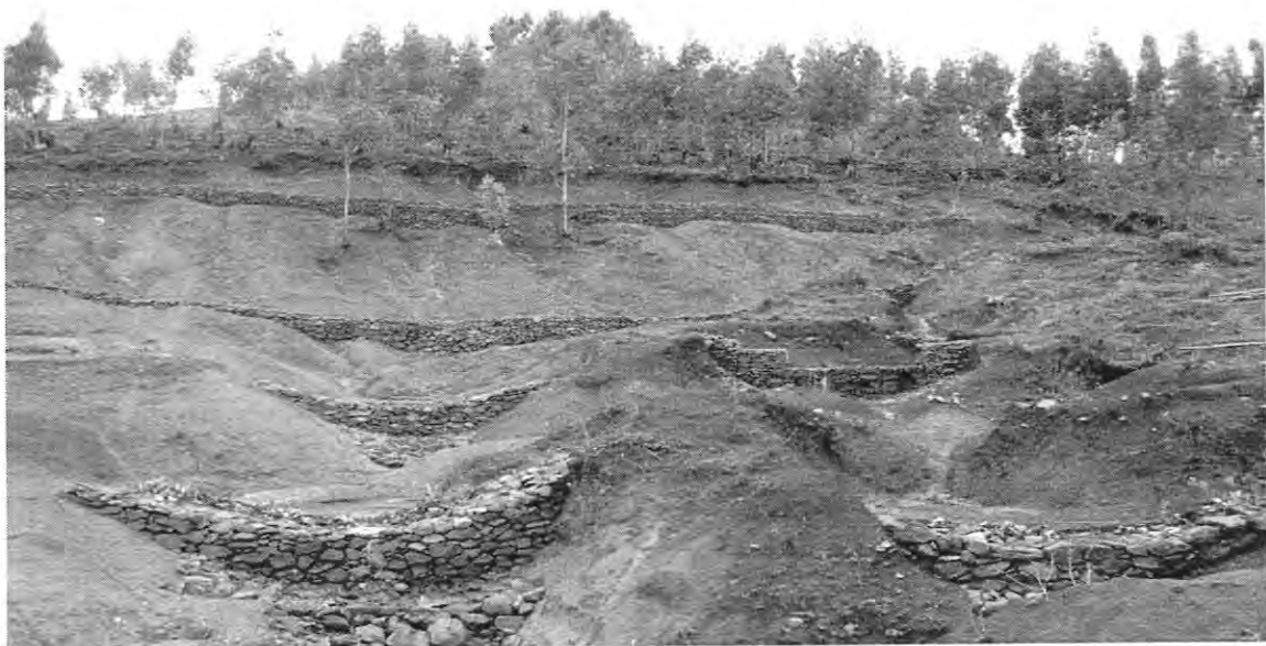
Figure 4. Check dams constructed on communal lands.
