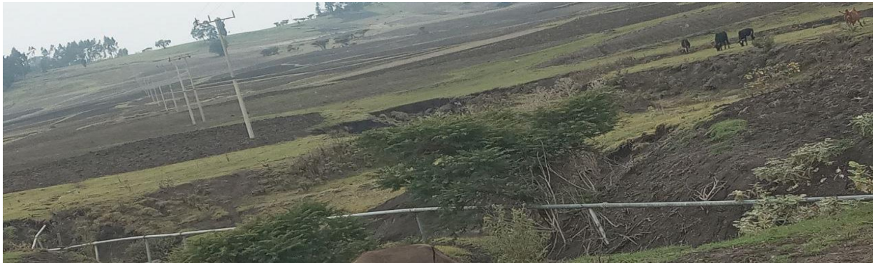
Figure 32: Photo of pipe installation taken during field survey
