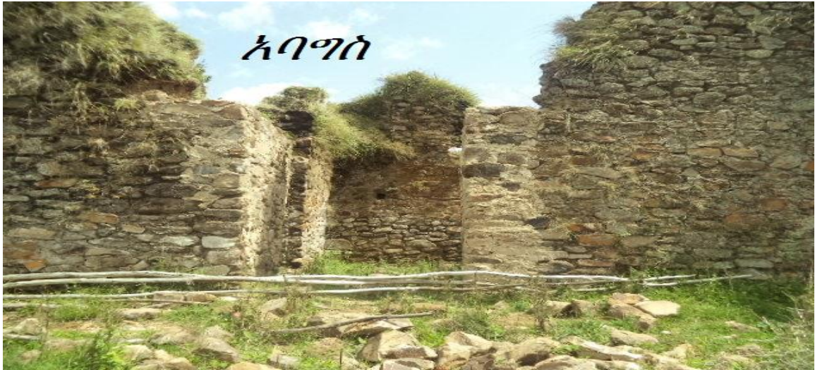
Figure 4.15:FASIL/ABA GIS/Ginb/ building
