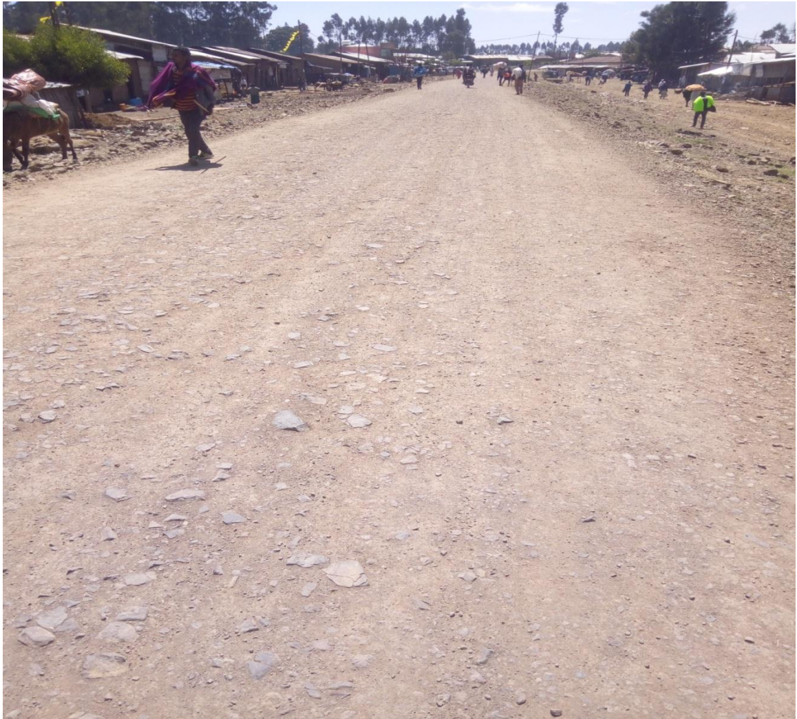
Figure 4.17: Service provider and road problems in Gish Abay Town
