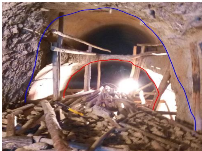
Plat 3.2 View of the outlet conduit during the construction
