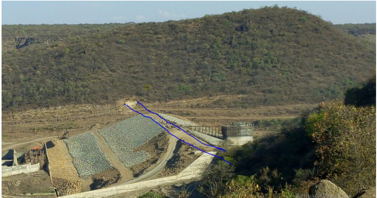
Plate 3.1 View of the dam from left side down stream
