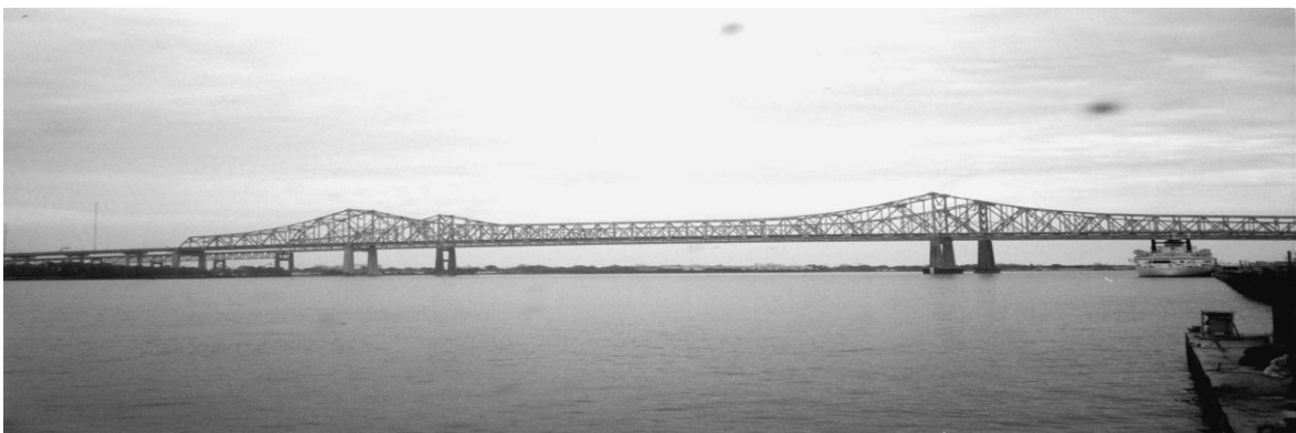
Figure 3.2 Through-Truss Bridge, Greater New Orleans Through-Truss Bridge (Courtesy of Amy Kohls, 1996.)
