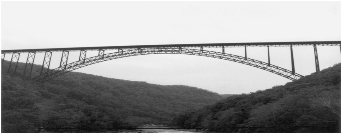
Figure 3.1 Truss-Arched Bridge, New River Gorge Bridge.(Courtesy of Michelle Rambo-Roddenberry, 1996.)
