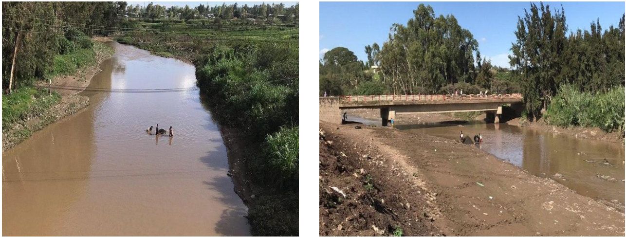
Figure 4-5 sand extraction below the new bridge at Tirunesh Beijing
