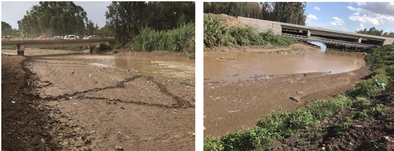
Figure 4-6 Sediment accumulation around Tirunesh Beijing bridge
