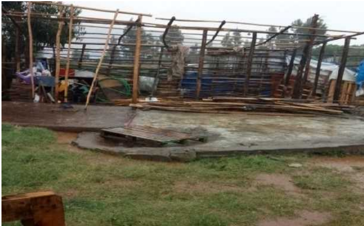
Fig 5. Squatter's house Demolished Source: Photo taken by the author, 2018
