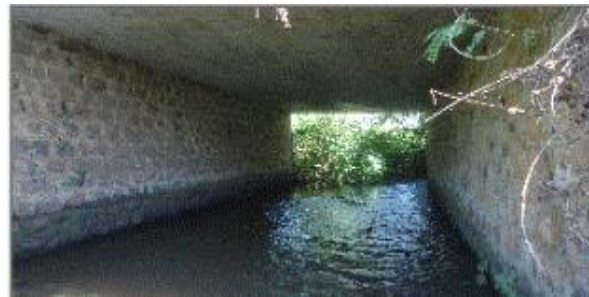
Fig 5.3 photo of Bitinwuha Bridge
