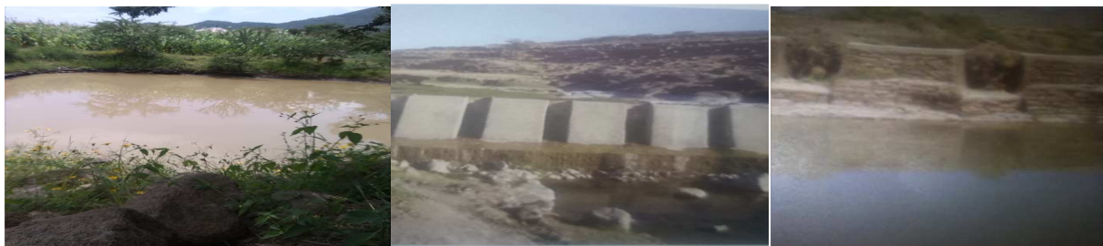
Figure27: Introduced water conservation structure
