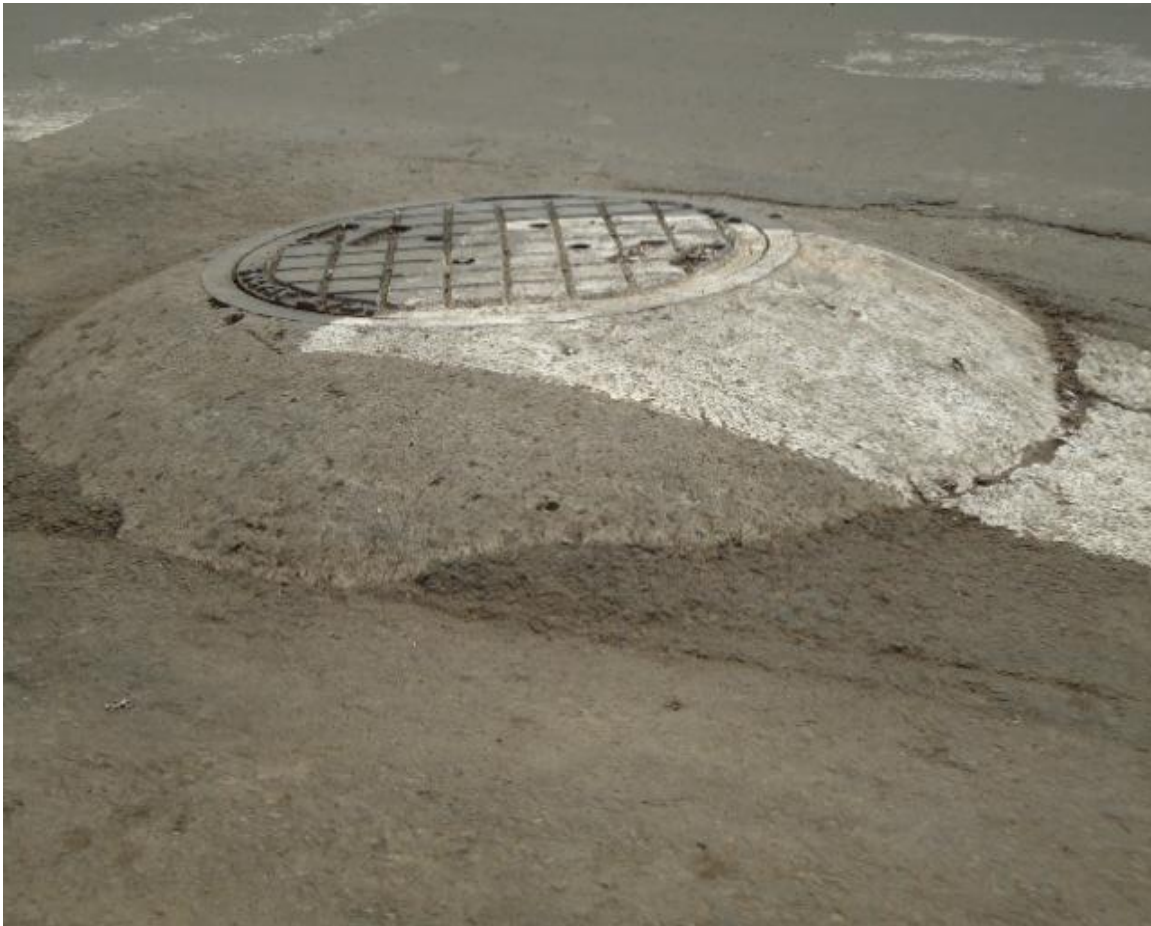
Figure 4.8: Sewer manhole around Casanches menharea area (Photo taken on june,2011)
