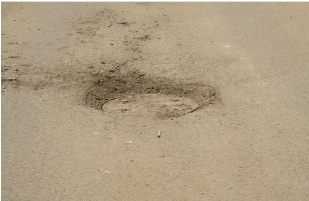
Figure 4.2 A sewer manhole around Berhanna Selam printing (Photo taken on June, 2011)
