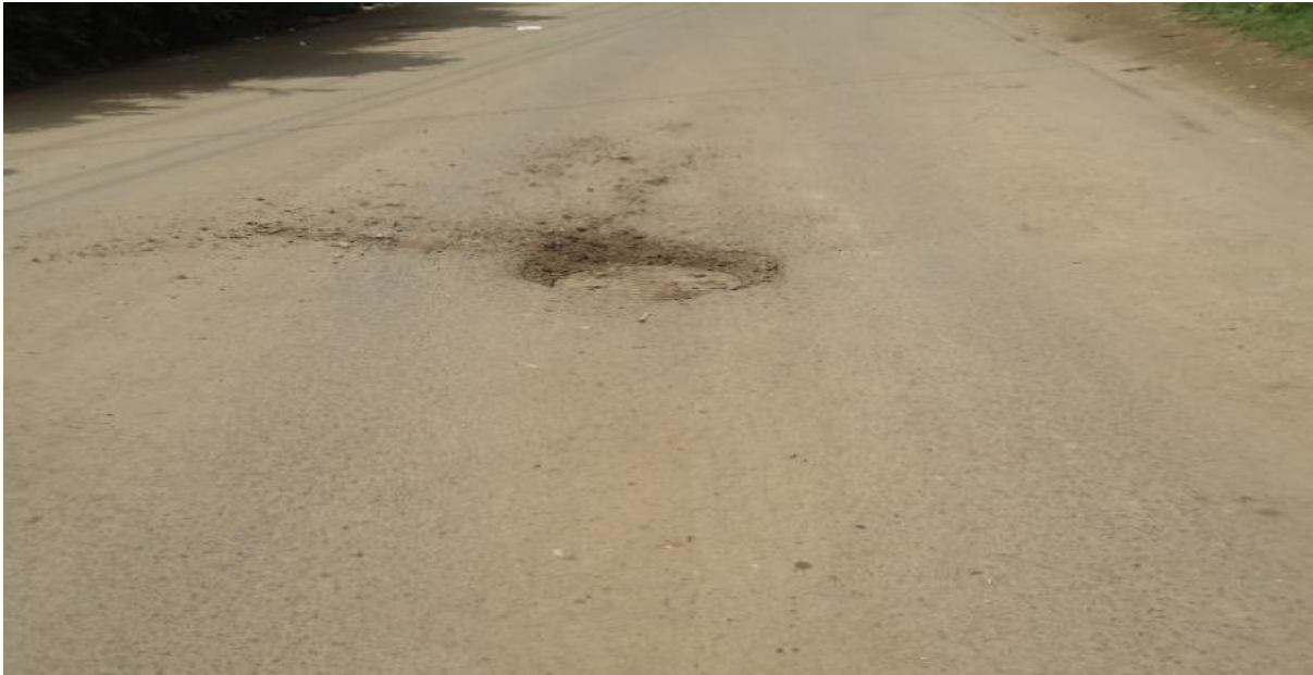
Figure 4.5: Sewer manhole around grand palace (Photo taken on June, 2011)
