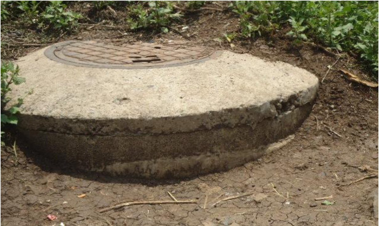
Figure 4.9: Sewer manhole around felweha area (Photo taken on June, 2011)
