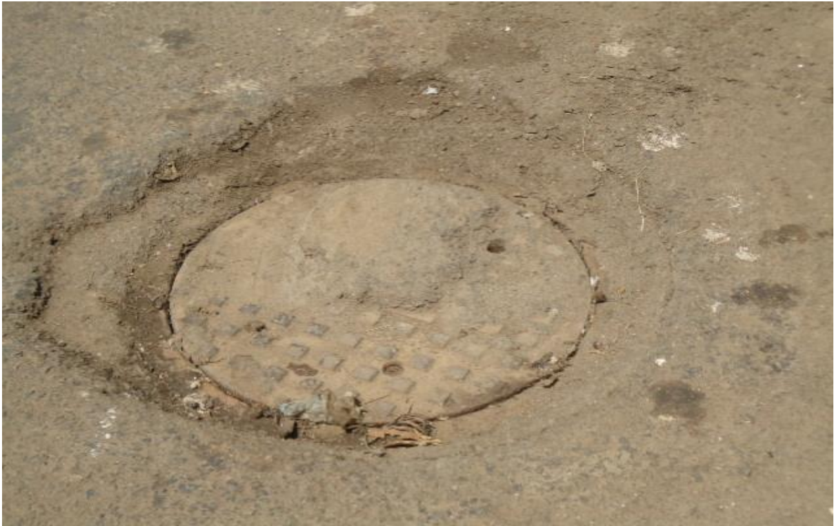
Figure 4.1: Sewer manhole around grand palace (Photo taken on June, 2011)
