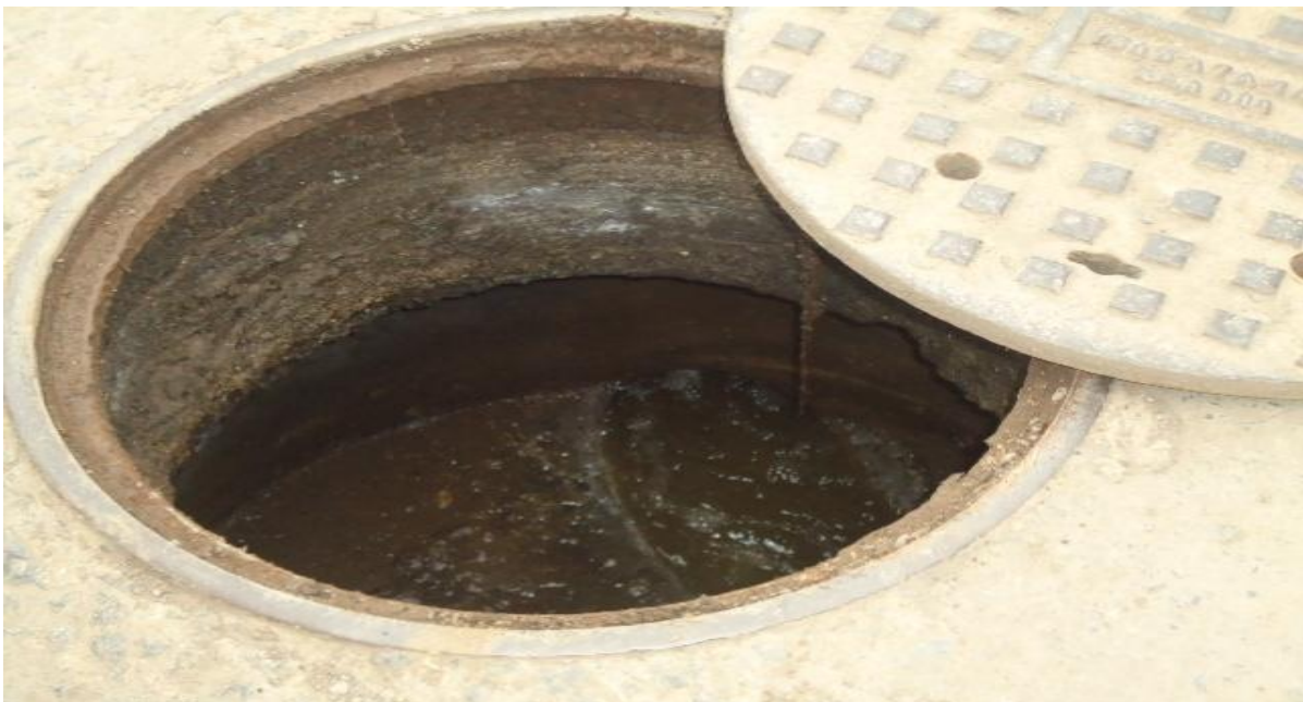
Figure 4.7 Sewer manhole around Zemen bank (Photo taken on June, 2011)
