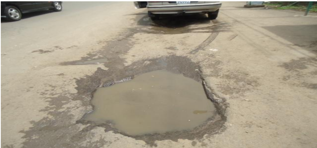
Figure 4.13: Sewer manhole around casanches (Photo taken on June, 2011)
