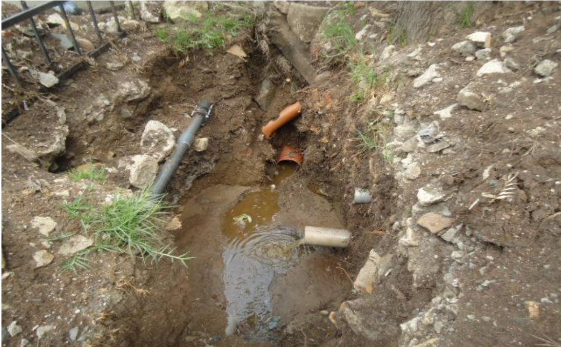
Figure 4.12: Sewer manhole around beside berhann selam printing (Photo taken on June, 2011)
