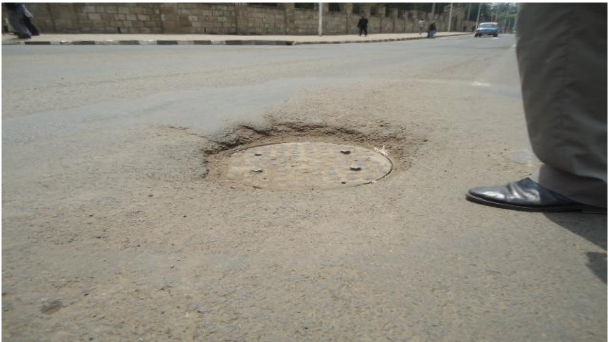
Figure 4.4 : Sewer Manhole around grand palace (Photo taken on june,2011)
