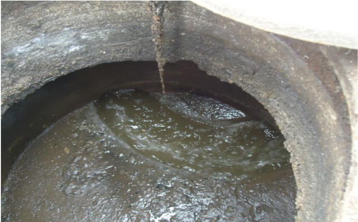
Figure 4.6 A sewer manhole around Zemen Bank (Photo taken on June, 2011)
